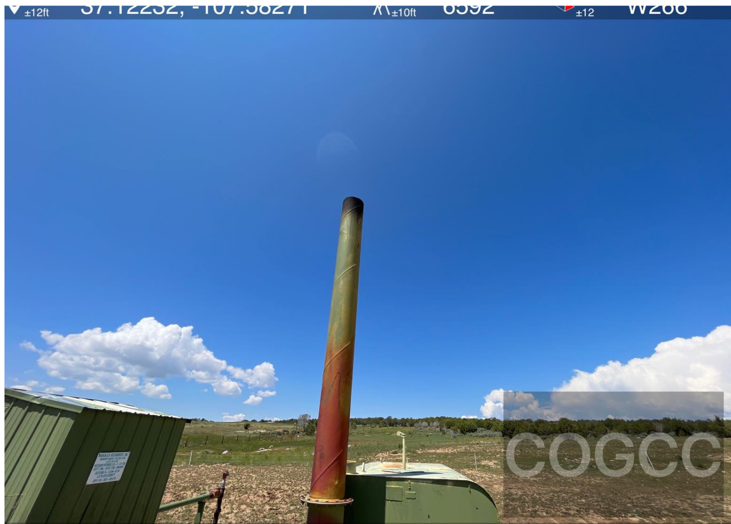
Photo #2 View of missing bird protection cap.
