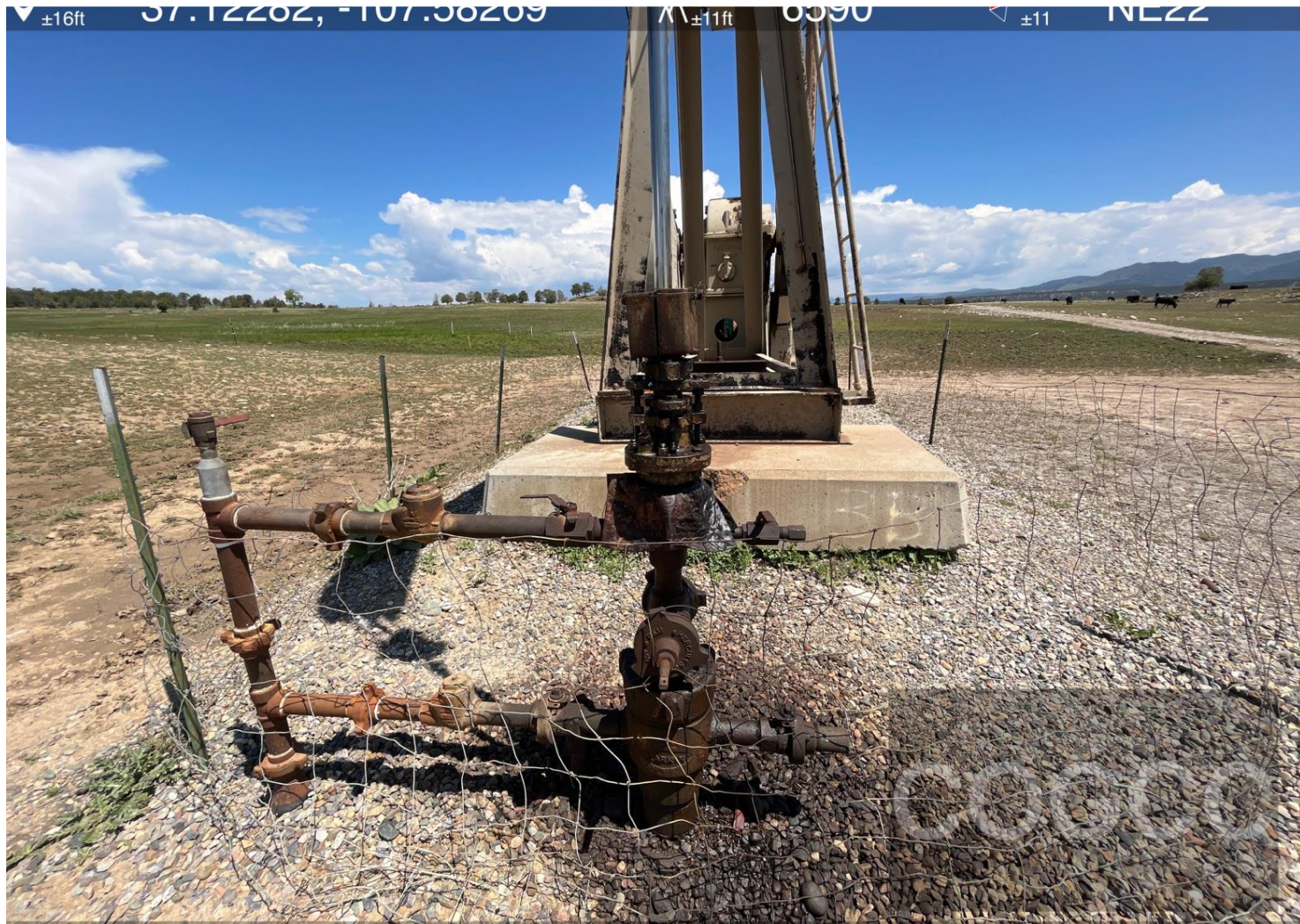
Photo #1 View of wellhead assembly and impacted material.
