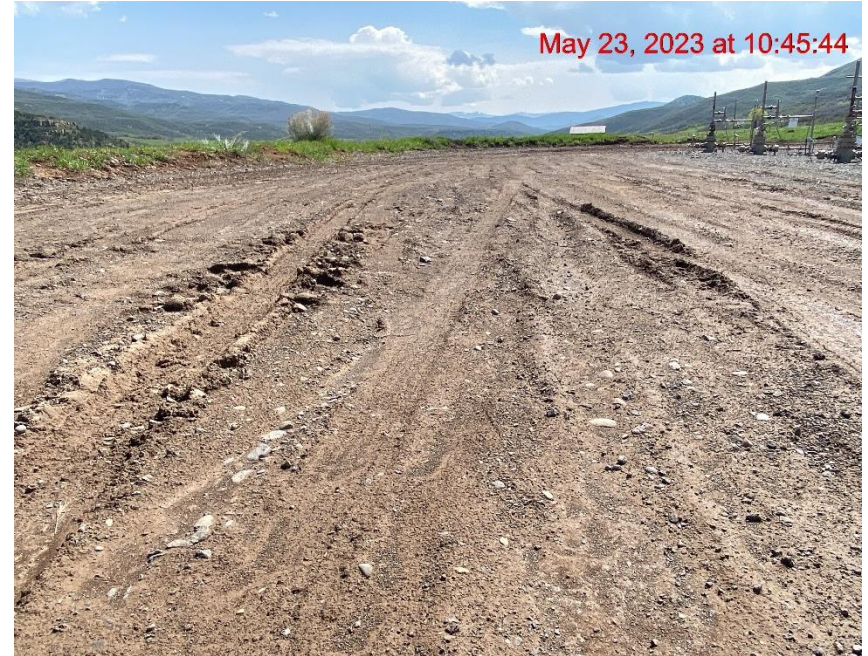
Location Lacks Stabilization – Photo #03726
