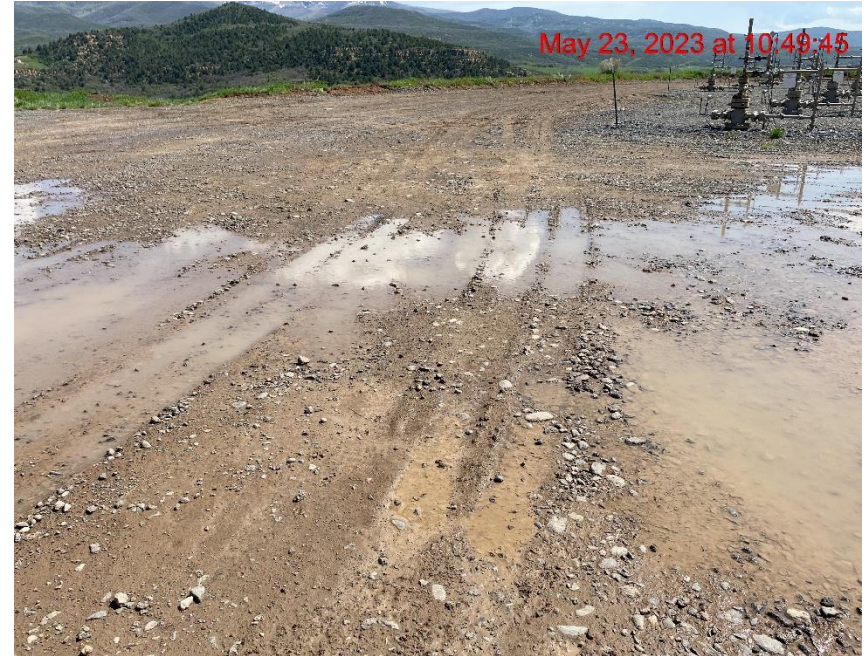
Location Lacks Stabilization – Photo #03732
