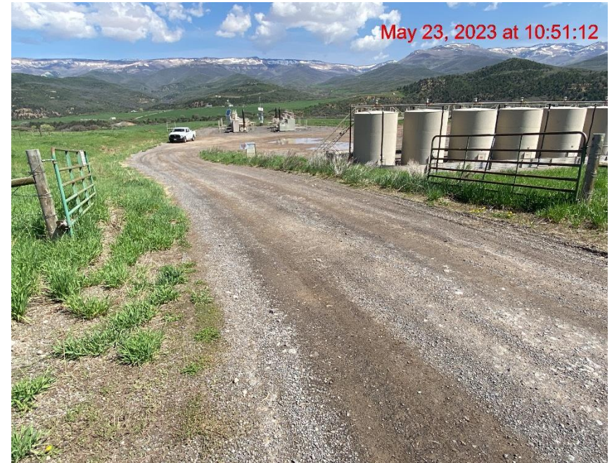
Insufficient Vehicle Tracking BMPs at Location Entrance/Exit – Photo #03735
