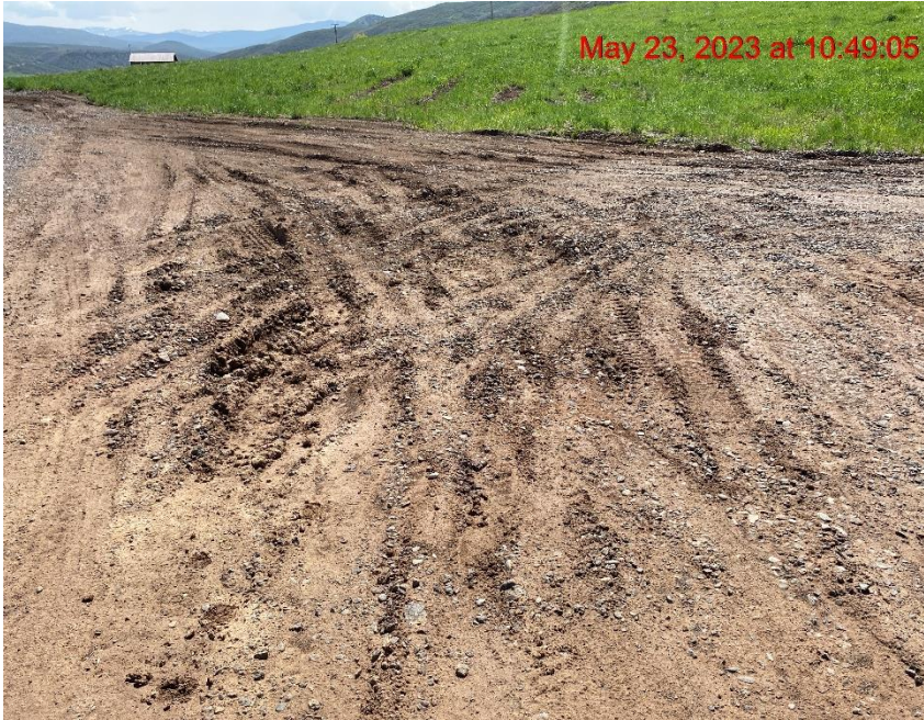
Location Lacks Stabilization – Photo #03731
