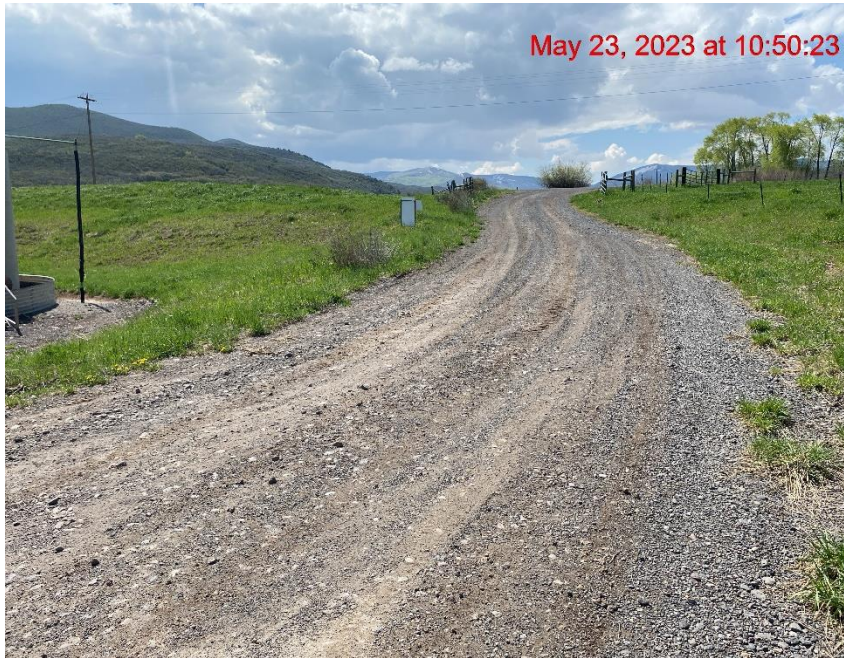
Insufficient Vehicle Tracking BMPs at Location Entrance/Exit – Photo #03734
