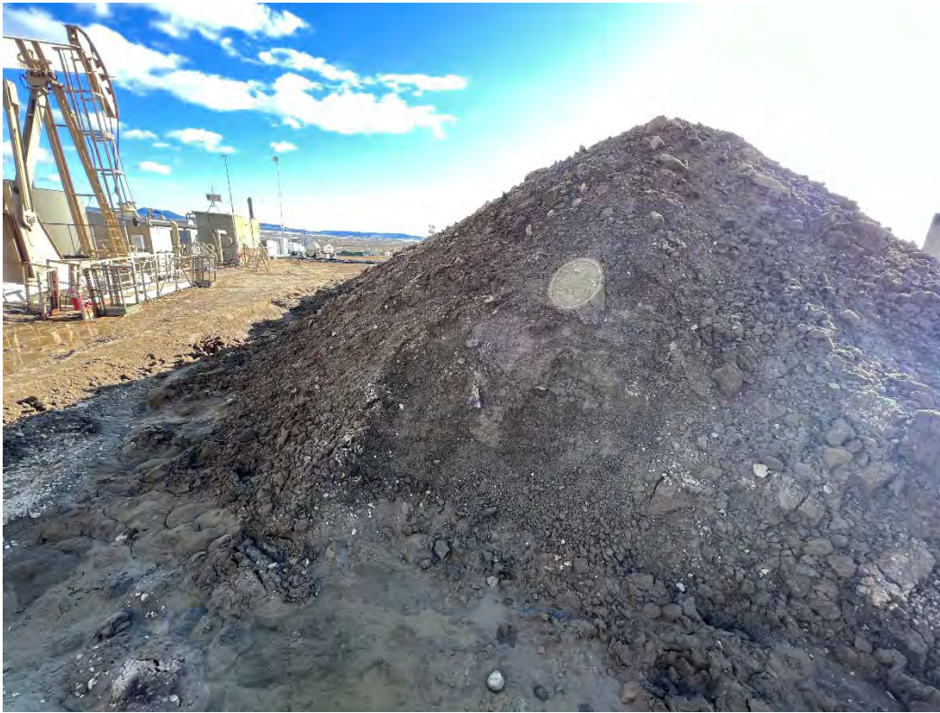
PHOTO NO 5: STOCKPILED CONTAMINATED SOIL PILE
