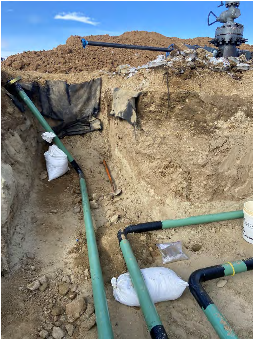
PHOTO No 9: SS_03 LOCATION. LOOKING NORTHWEST.
