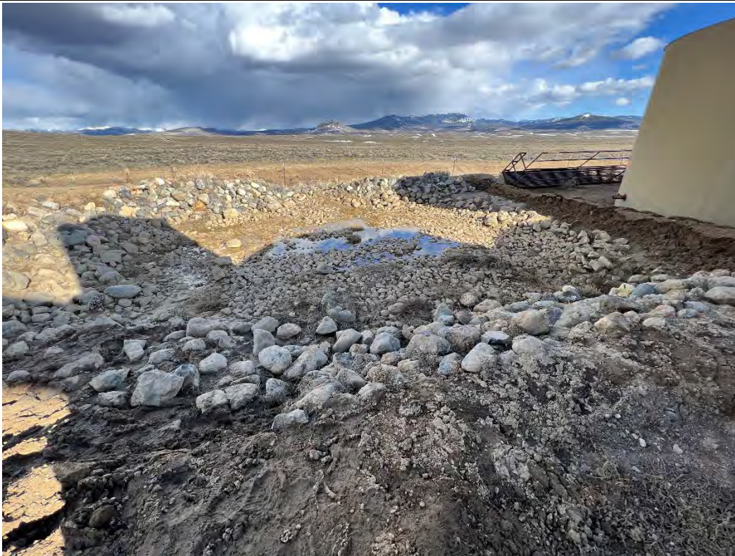
PHOTO NO 6: STORMWATER RETENTION BASIN
