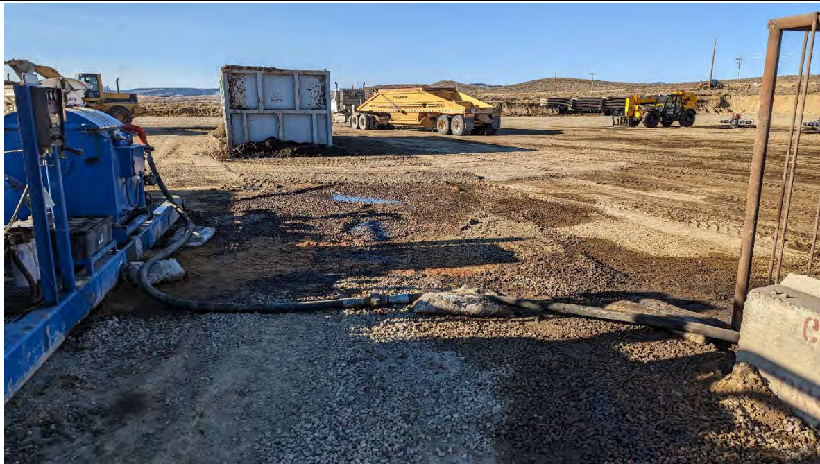
PHOTO NO 12: PAD FACING SOUTHWEST FROM NORTHEAST CENTRAL PAD.
