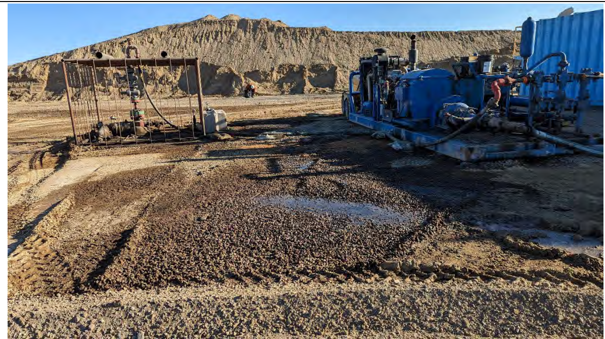
PHOTO No 6: PAD FACING NORTHEAST FROM CENTER OF PAD.
