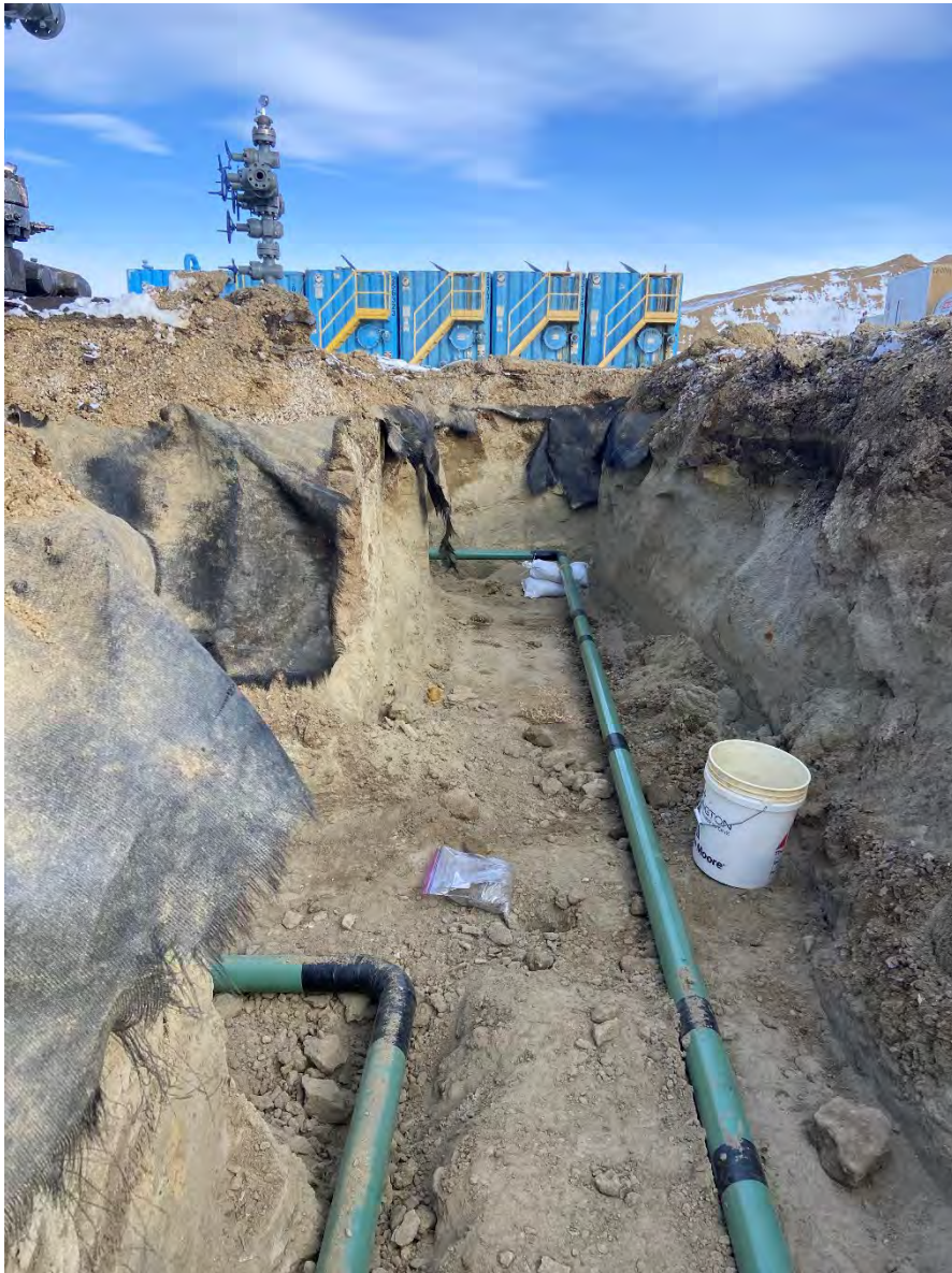
PHOTO No 8: SS_02 LOCATION. LOOKING NORTHEAST.
