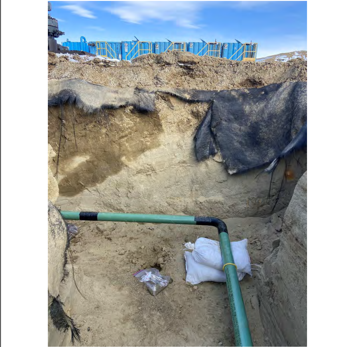
PHOTO No 7: SS_01 LOCATION. LOOKING NORTHEAST.
