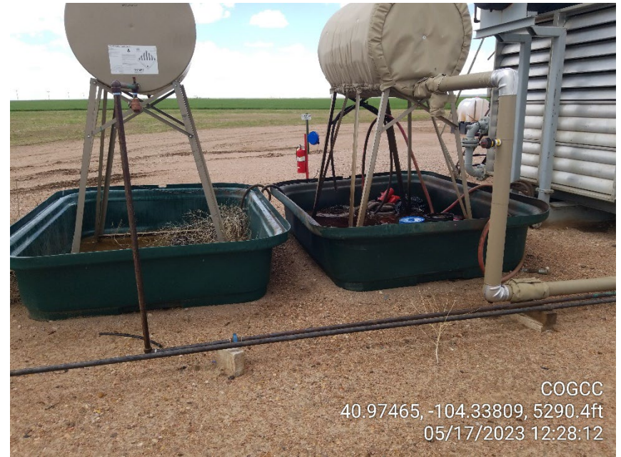
Photo 10 – Wildlife Nettings are in disrepair – Debris and Oily Waste
