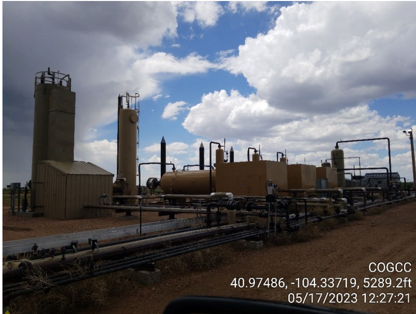
Photo 7 – Separators and Heater Treaters
