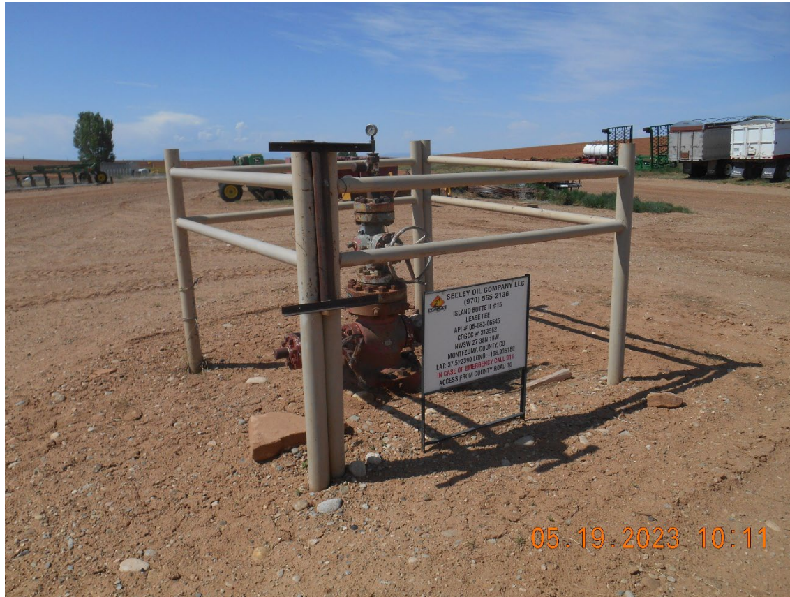
Injection Wellhead – Temporarily Abandoned
