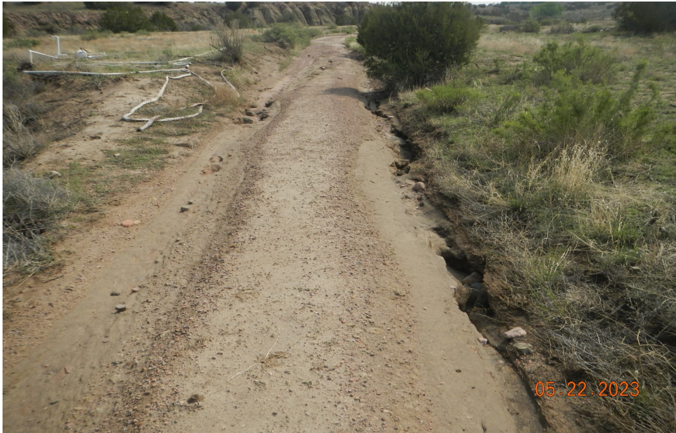
Photo 9. Facing northeast along the access road near the location. Stormwater has caused an erosion channel along the road that needs to be repaired.
