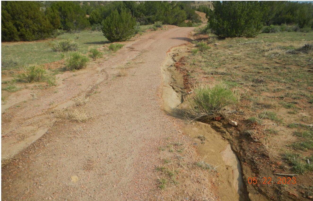
Photo 2. Facing northwest further along the access road. A recent storm event has created an erosion channel down the road which needs to be repaired.
