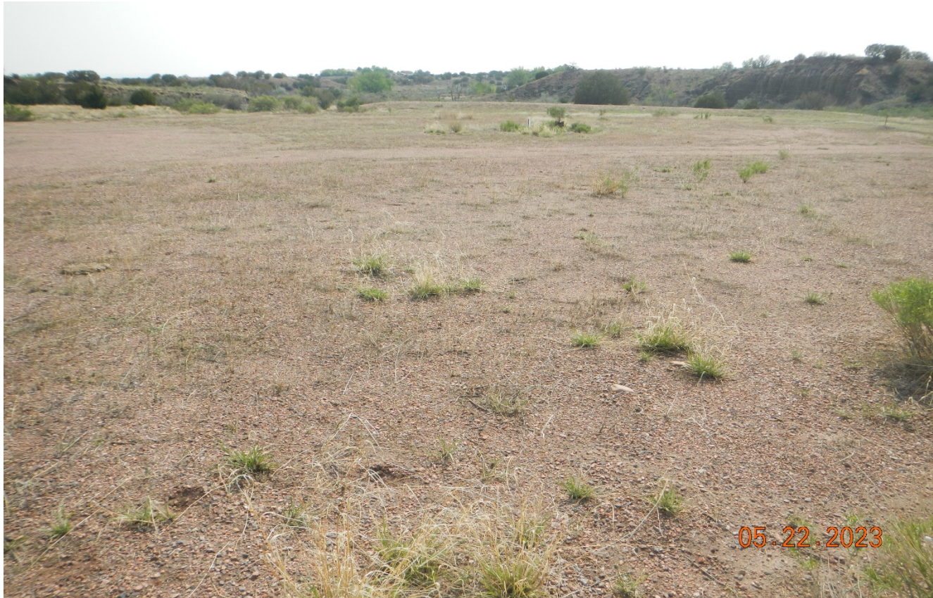
Photo 16. Southwest side of the location facing northeast. The location is not reclaimed and needs to be reduced in size. Gravel remains along unused areas of the location.
