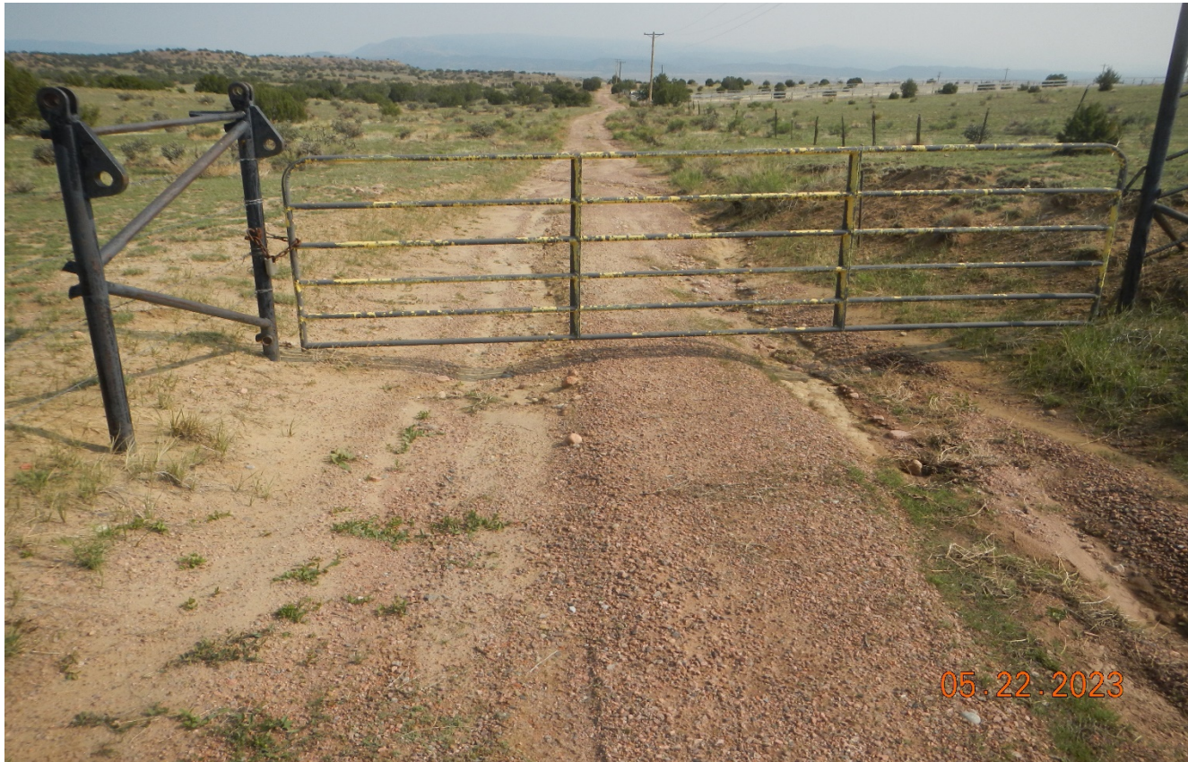
Photo 1. Facing north along the access road. There is erosion that has occurred along the road that needs to be repaired and stabilized.
