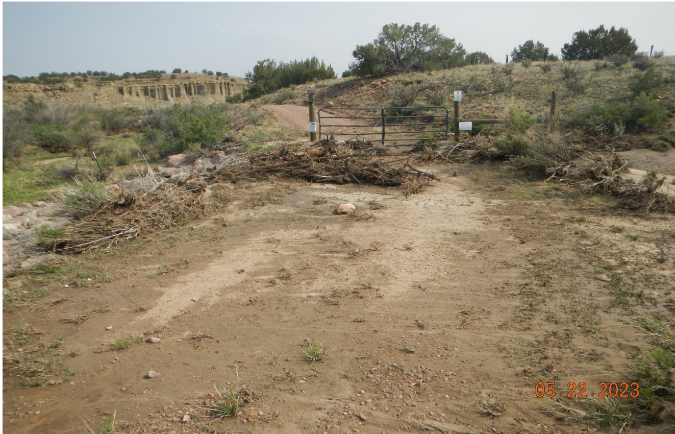
Photo 7. Further north along the access road at the second drainage crossing. Stormwater flowed over the culvert in this area which washed up debris in this area that will need to be cleaned up and removed.
