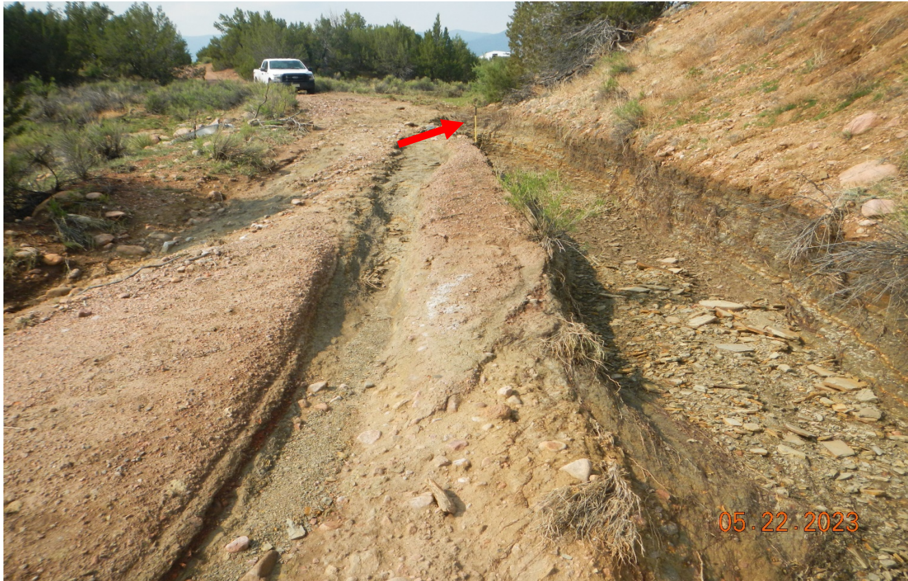
Photo 6. Facing back to the area of the road that has been washed out. Red arrow points to the shovel shown in the same place as previous photo.
