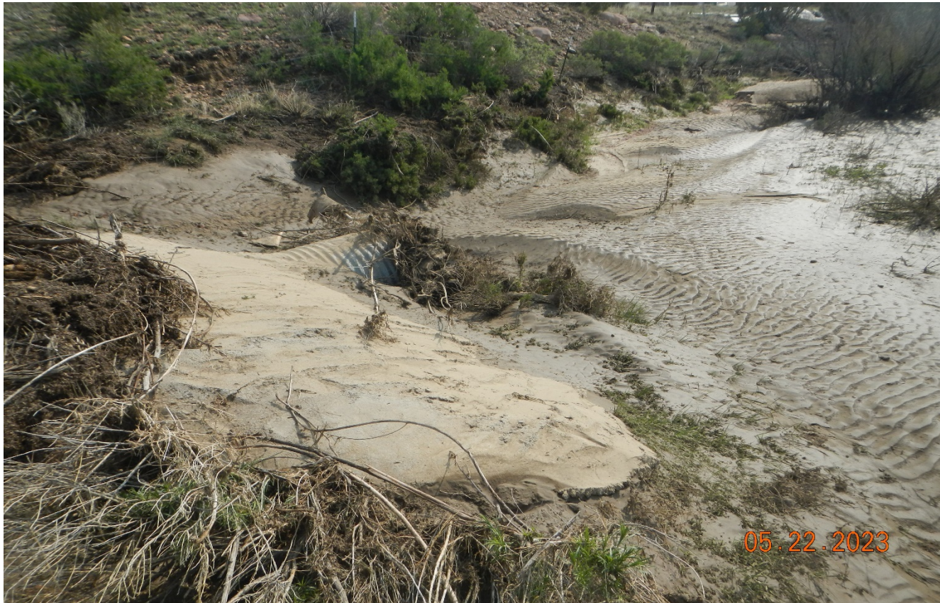
Photo 8. The culvert at this drainage crossing has filled in with sediment and debris.
