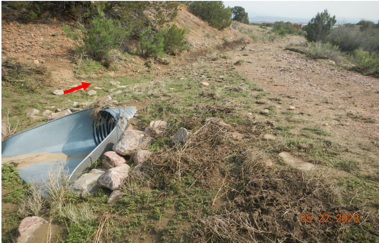
Photo 4. Facing toward the culvert at the drainage crossing. The recent storm event directed stormwater past the culvert at the red arrow causing erosion further down the road shown in the next photo.
