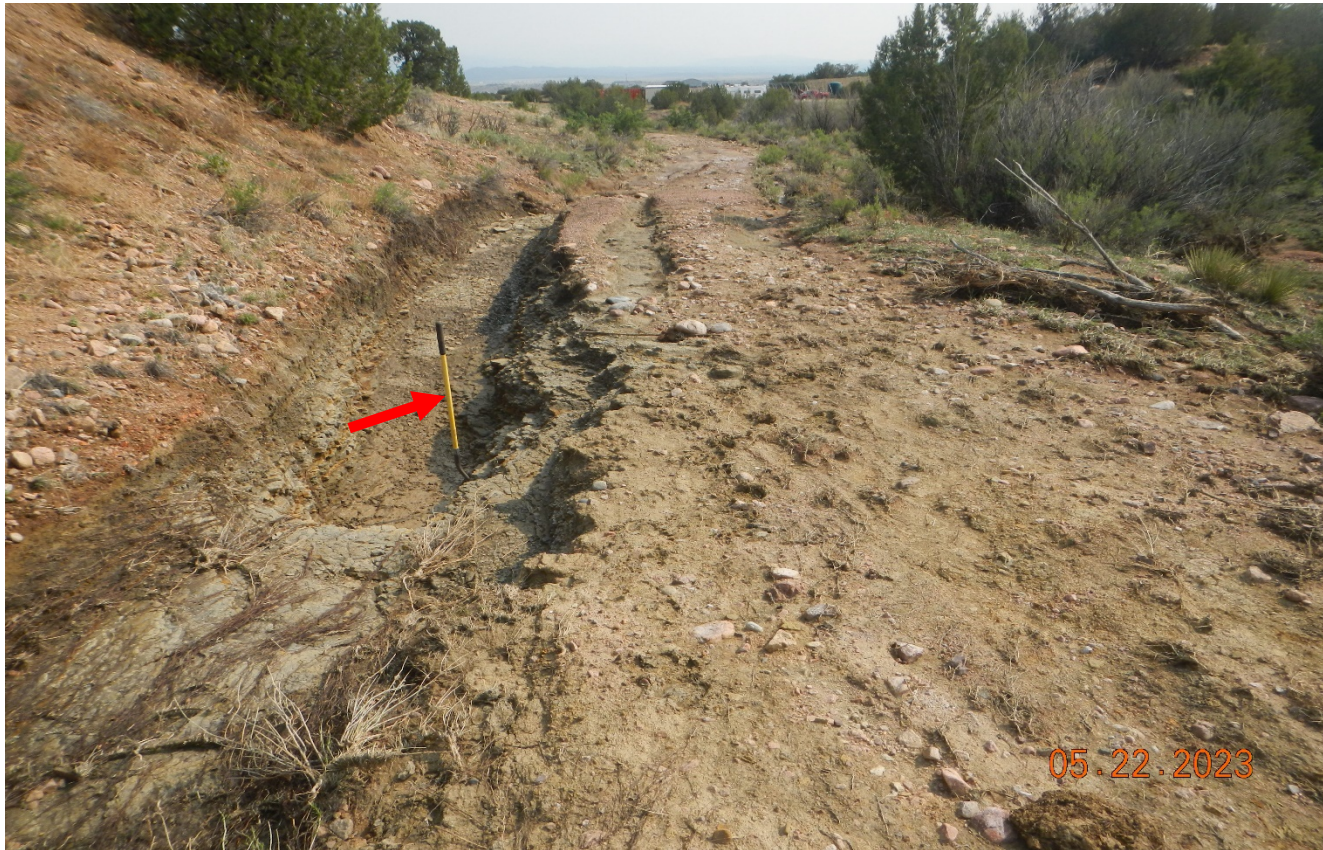
Photo 5. There was significant erosion of the road that occurred from the recent storm event. There is an approximate 4' gully along the road side in this area. Red arrow points to 4.5 ft. shovel placed in the gully.
