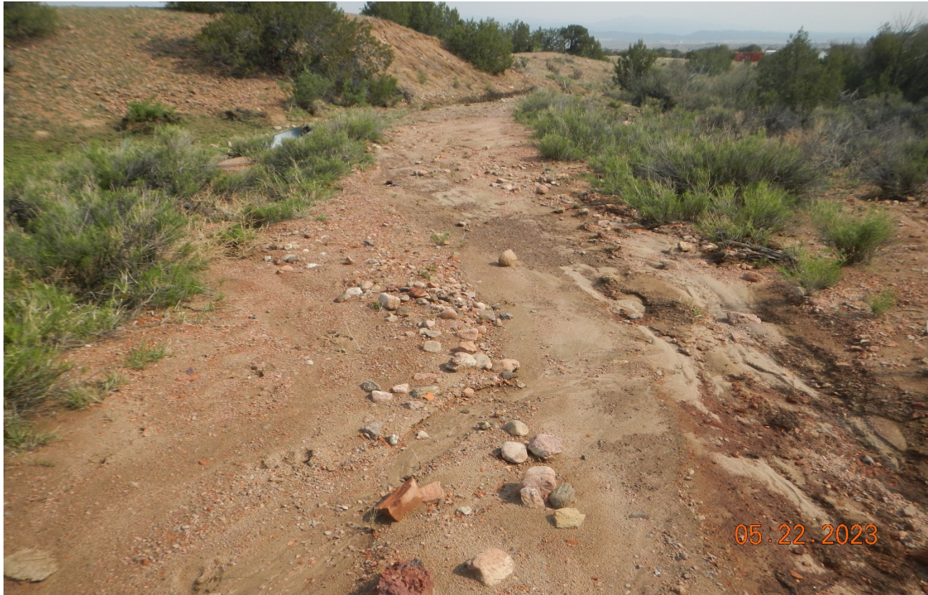
Photo 3. Facing north at the drainage crossing along the road. Stormwater has caused erosion of the road and has washed gravel and sediment off the road.
