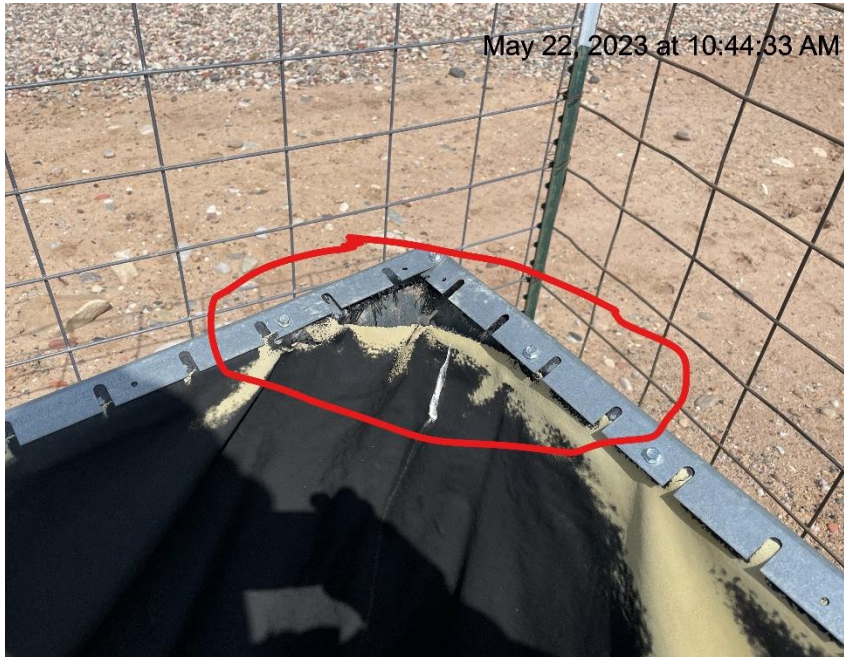
Photo # 8328 Containment liner needs maintenance
