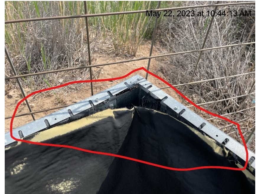
Photo # 8327 Containment liner needs maintenance
