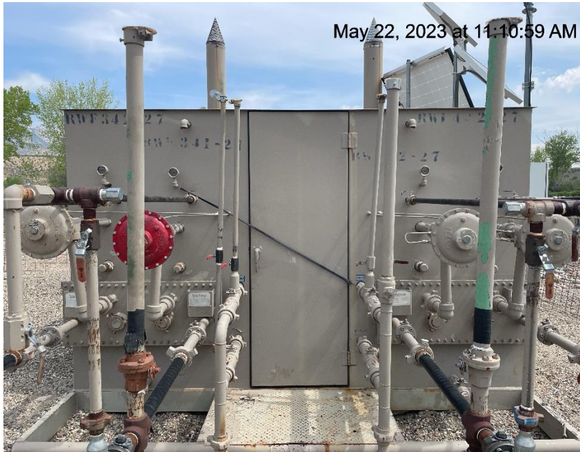
Photo # 8357 Meter calibration info not conspicuously posted
