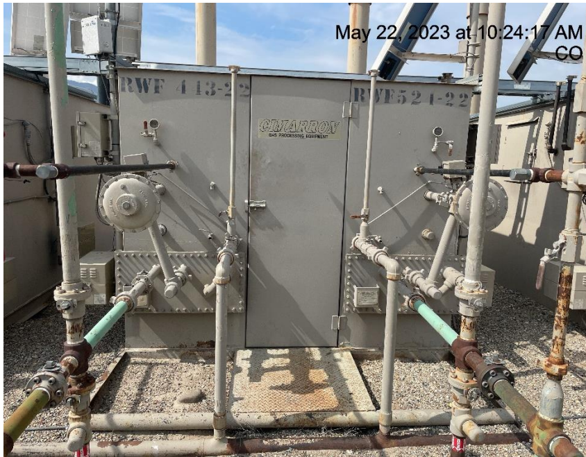
Photo # 8307 Meter calibration info not conspicuously posted
