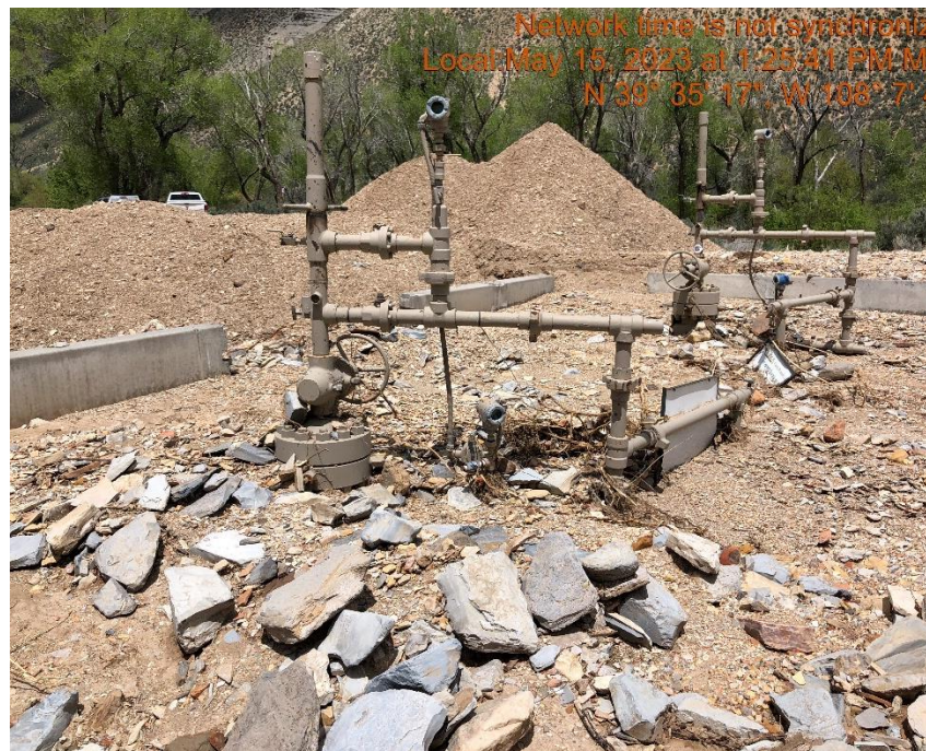
Photo #17 Wellheads inundated with sediment.
