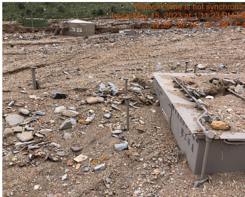
Photo #9995 Separator inundated with sediment.
