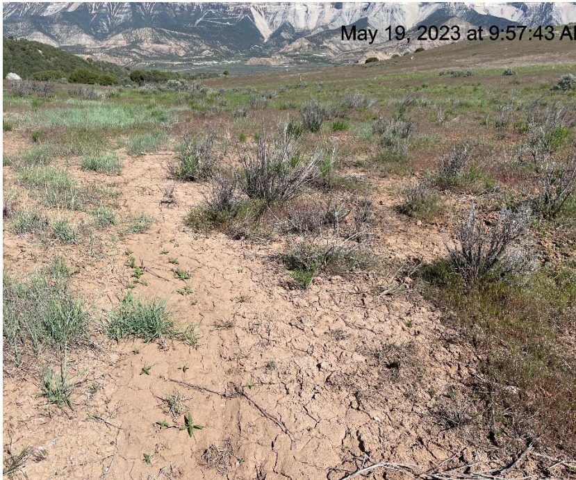
Photo # 8228 Erosion & transport of sediment off location into vegetation/insufficient BMP's (NW corner of location)
