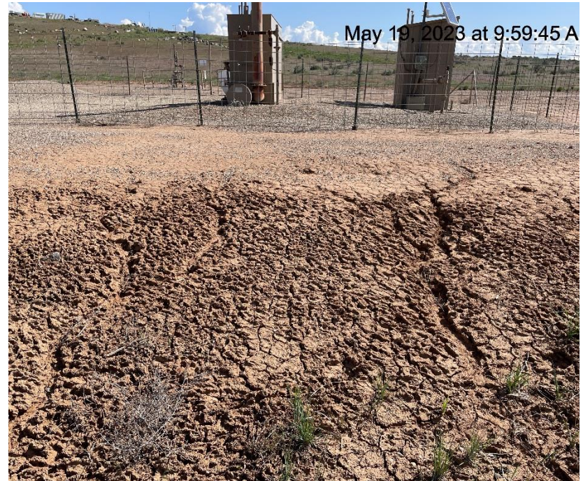
Photo # 8233 Erosion & transport of sediment off location into vegetation/insufficient BMP's (South side of location)
