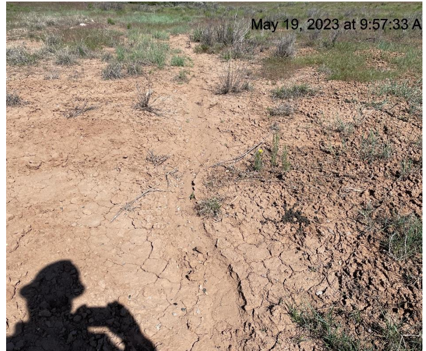
Photo # 8227 Erosion & transport of sediment off location into vegetation/insufficient BMP's (NW corner of location)
