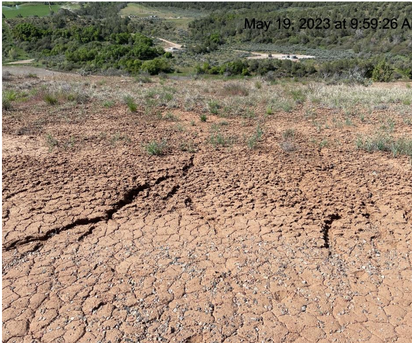
Photo # 8232 Erosion & transport of sediment off location into vegetation/insufficient BMP's (South side of location)
