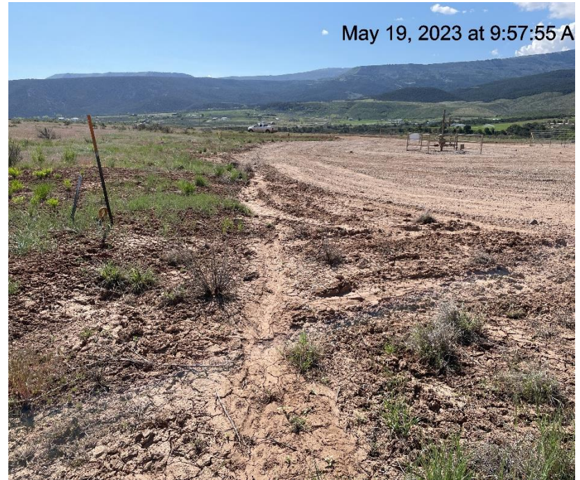
Photo # 8229 Erosion & transport of sediment off location into vegetation/insufficient BMP's (NW corner of location)
