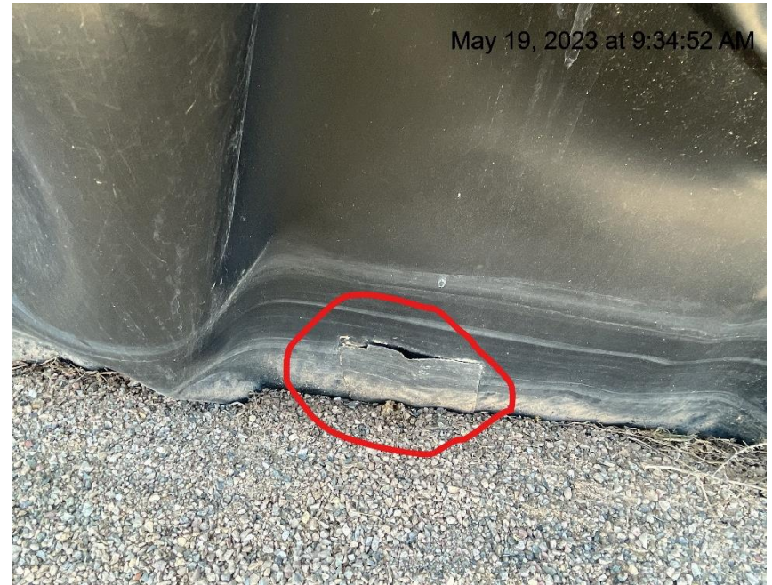
Photo # 8201 Containment liner needs maintenance
