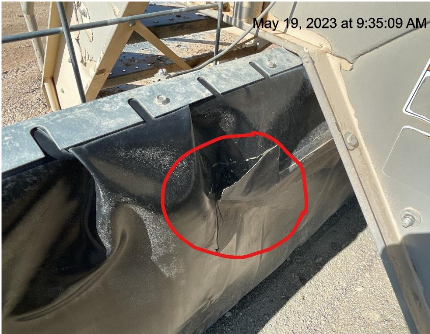
Photo # 8202 Containment liner needs maintenance
