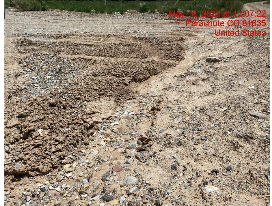
Rill Erosion Transporting Sediment Across Access Road Entrance – Photo #03525
