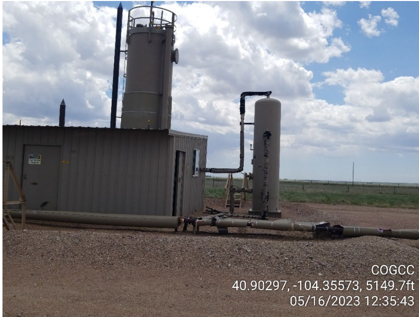
Photo 3 – Heater Treater
