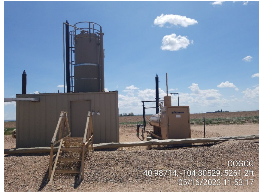
Photo 4 – Heater Treater and Separator
