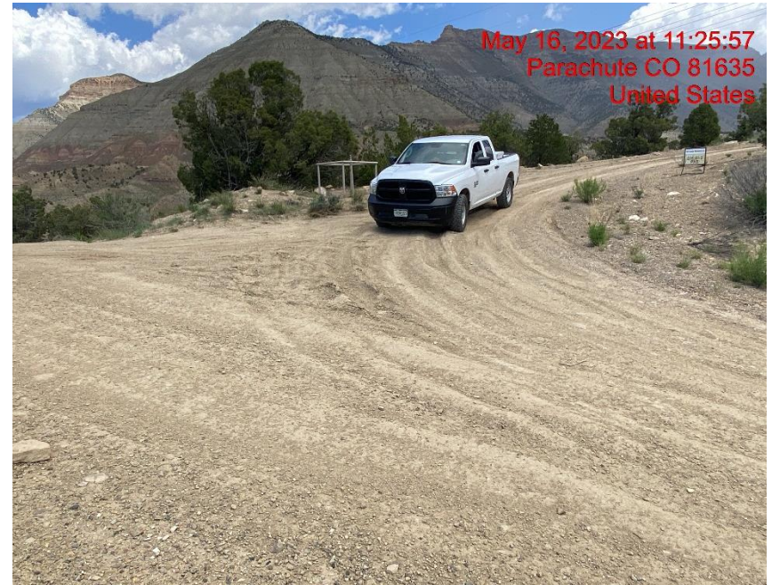
Insufficient Vehicle Tracking BMPs at Location Entrance/Exit – Photo #03441
