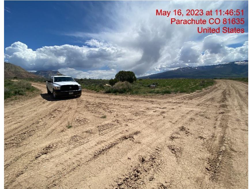
Insufficient Vehicle Tracking BMPs at Location Entrance/Exit – Photo #03479
