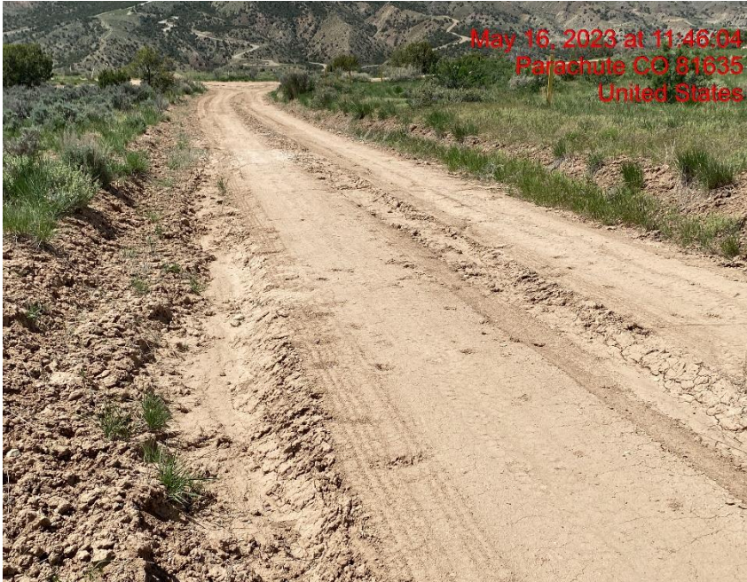
Access Road Degradation/Transportation of Sediment – Photo #03478
