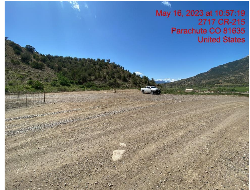
Insufficient Vehicle Tracking BMPs at Location Entrance/Exit – Photo #03396
