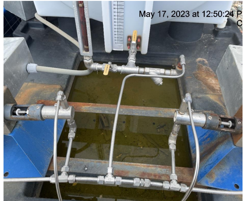
Photo # 7974 Chemical containment full of fluid/Failure to maintain chemical BMP
