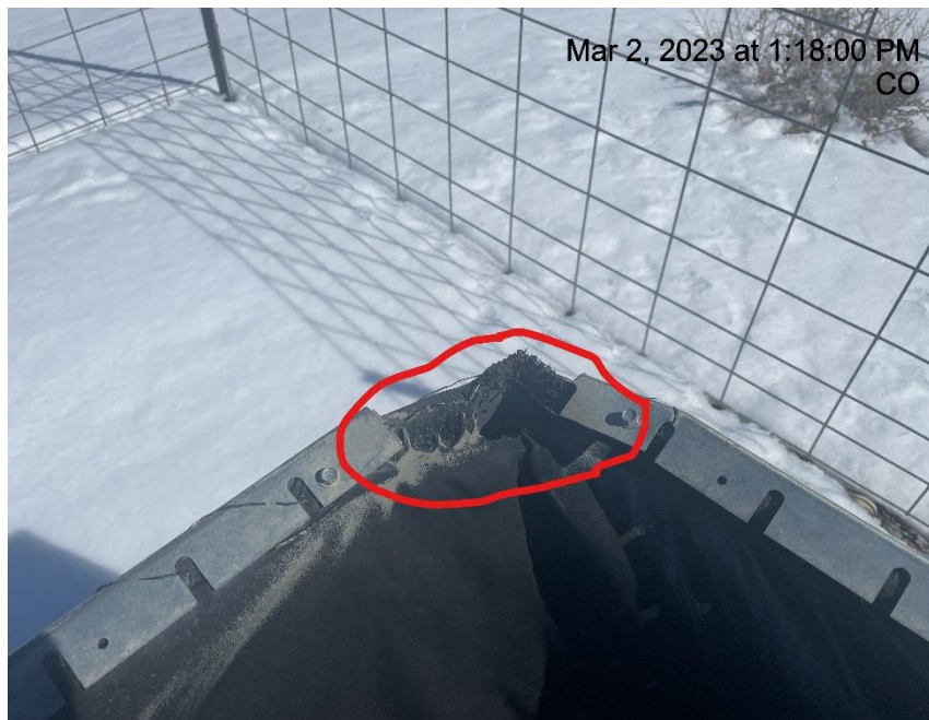
Photo # 1511 From inspection 708900066 conducted on 03/02/2023 Containment needs maintenance
