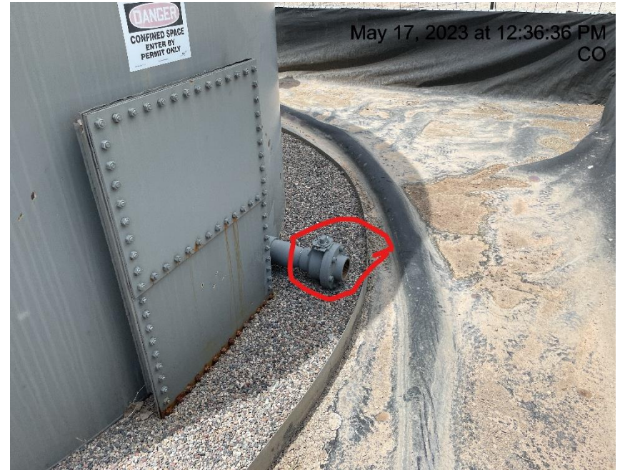
Photo # 7934 Open ended load line
