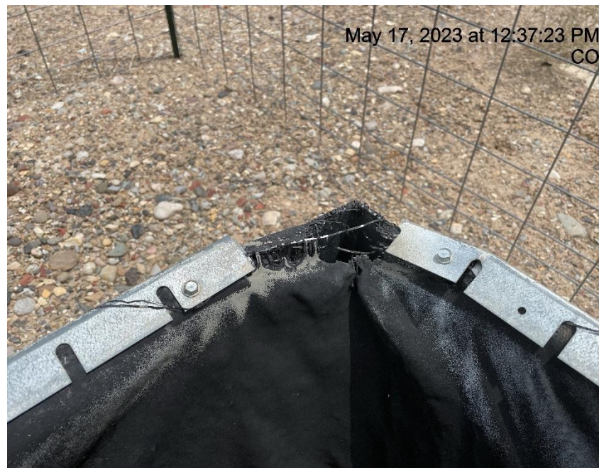
Photo # 7937 Containment needs maintenance
