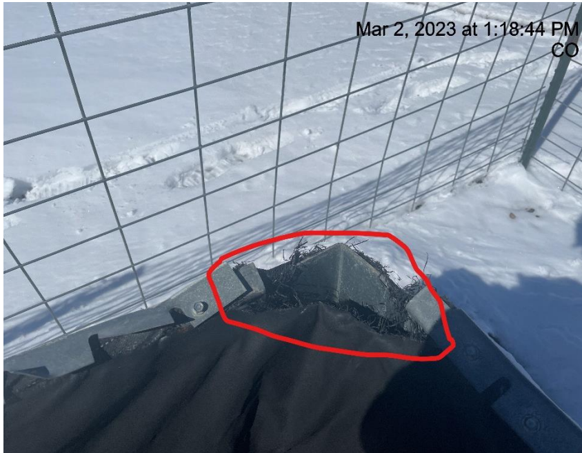
Photo # 1514 From inspection 708900066 conducted on 03/02/2023 Containment needs maintenance
