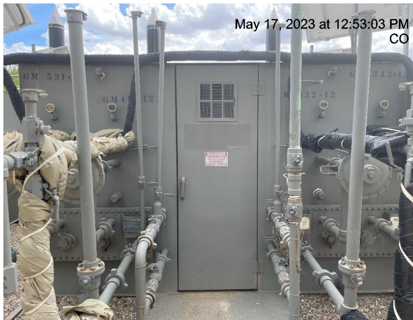
Photo # 7977 Meter calibration info not conspicuously posted
