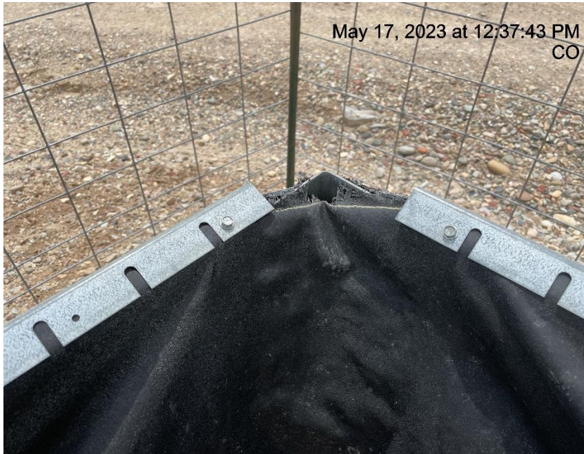
Photo # 7938 Containment needs maintenance
