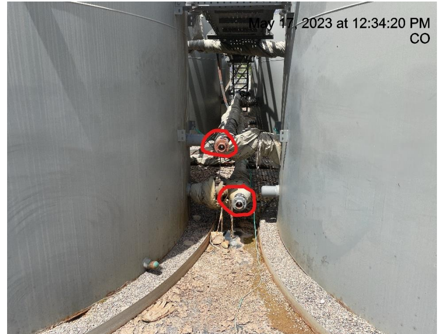
Photo # 7930 Open ended load lines
