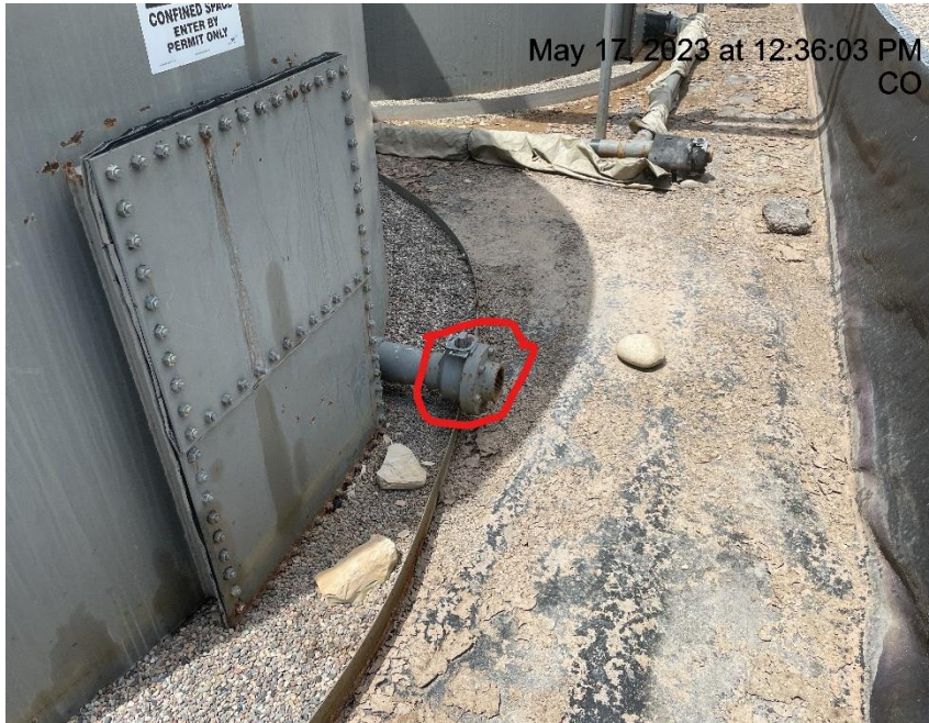
Photo # 7931 Open ended load line
