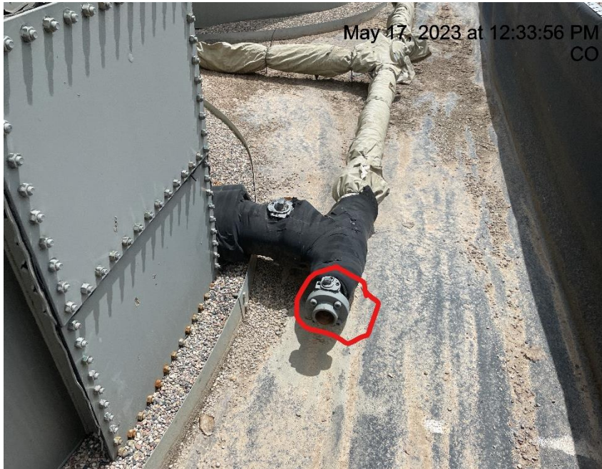
Photo # 7929 Open ended load line
