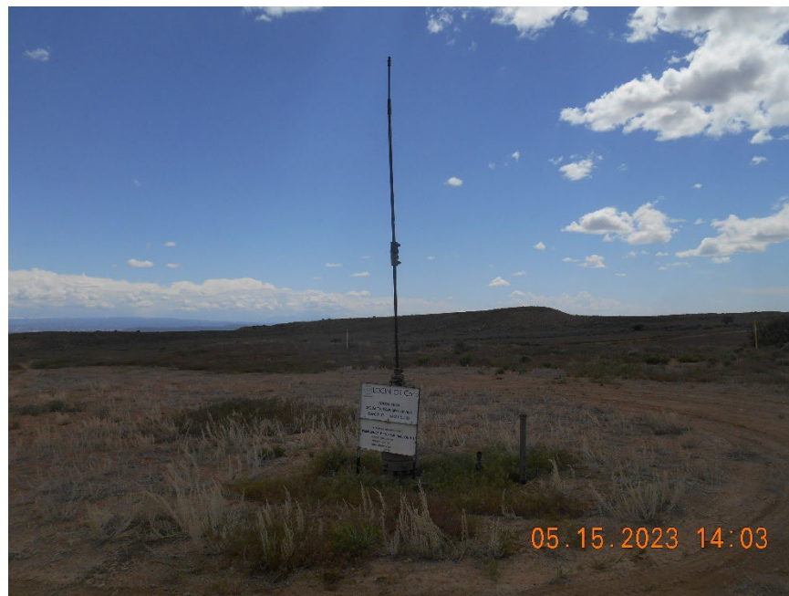
Wellhead with sign.
