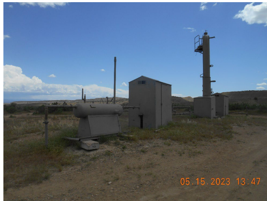
Separator, Meter housings and Dehydrator
