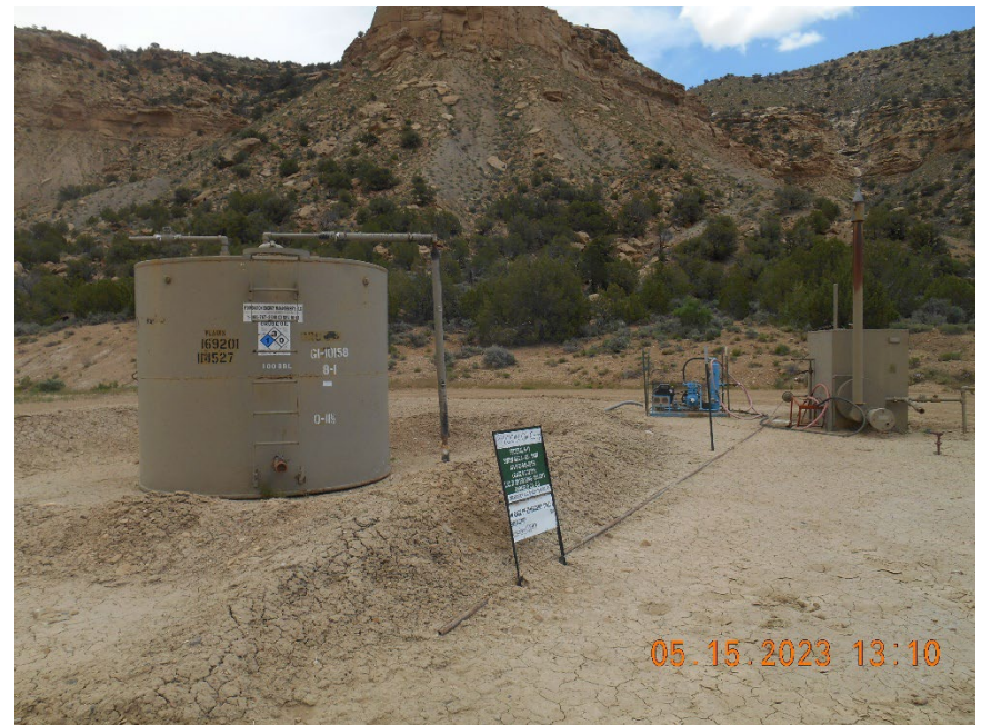
Tank Battery, Separator and compressor
