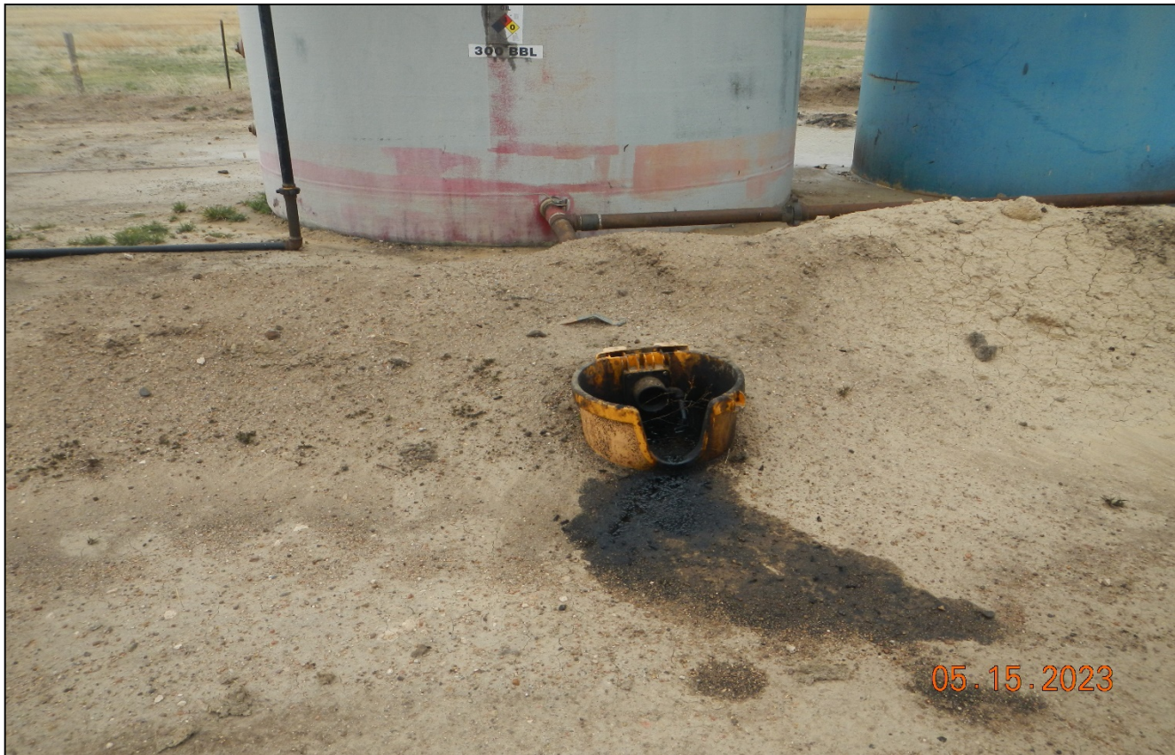
Photo 2. There is oil stained soils at the tank outlet that need to be cleaned up. The containment cover needs to be repaired.
