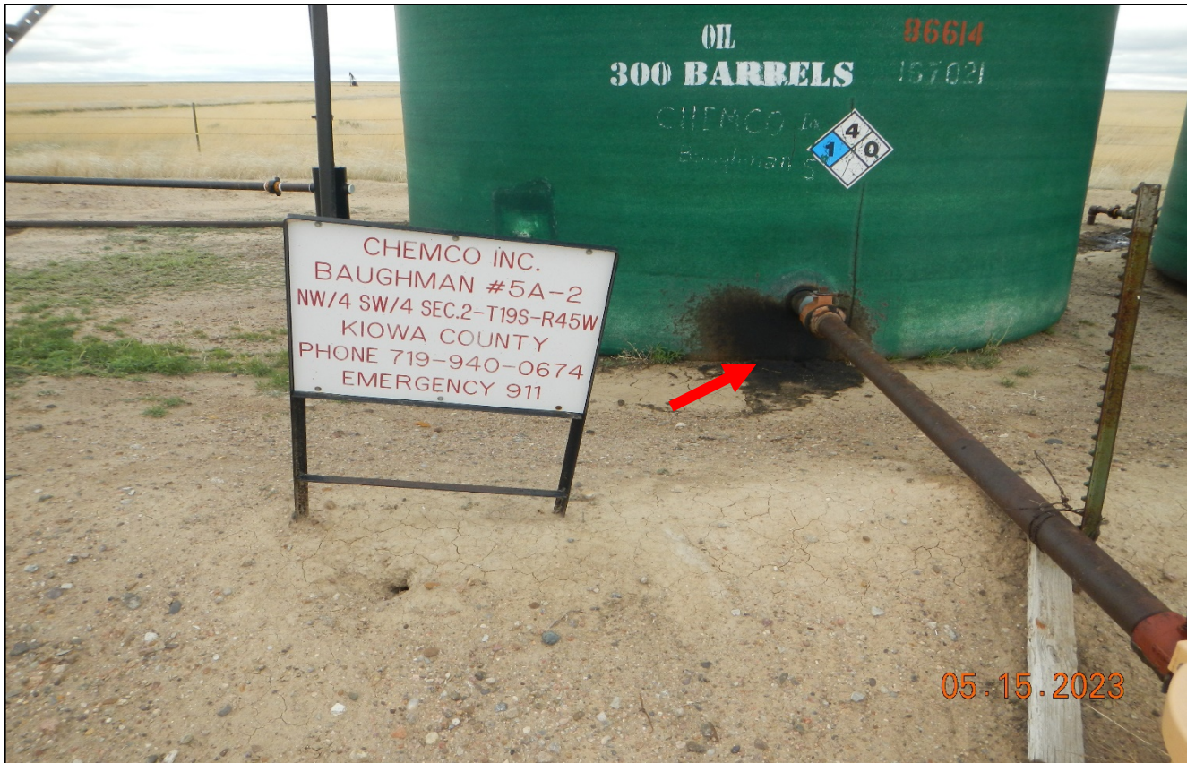
Photo 2. Sign is posted at tank battery. There is a leak and stained soils shown at red arrow.
