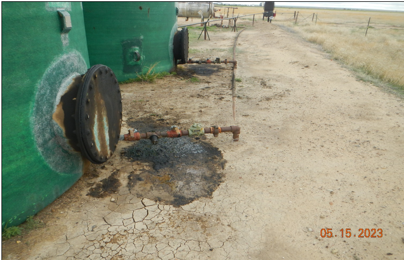
Photo 3. There is a leak at the pipe outlets at the backside of the tanks. Stained soils need to be cleaned up and leak needs to be repaired.
