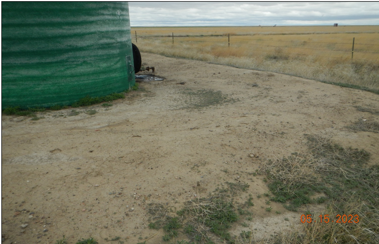
Photo 4. The berms around the tanks are insufficient to contain a spill.
