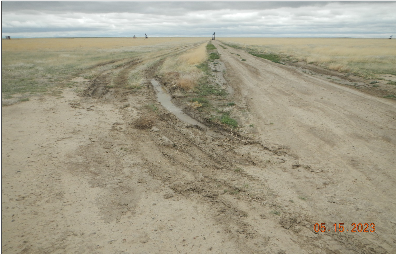
Photo 6. Facing east along the access road to the wellsite. Vehicles are driving outside of the designated road boundary causing unnecessary disturbance which will need to be reclaimed.
