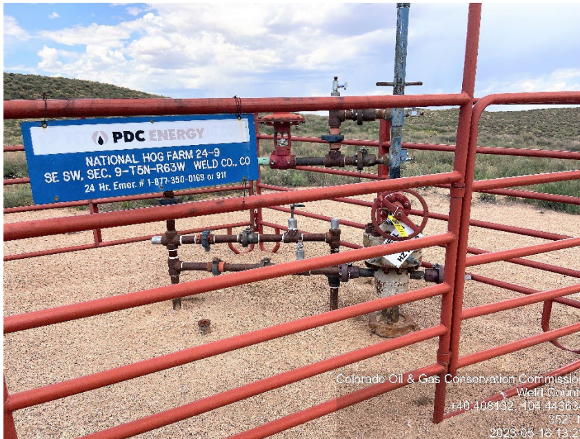
Photo #1 NHF 24-9 (123-20923) Wellsite Temporarily Abandoned | TA
