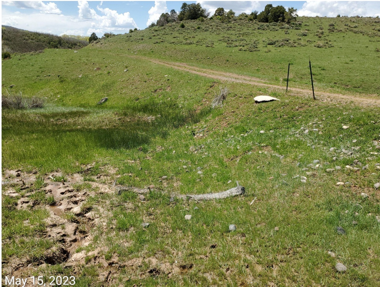
Photo 9: Photo shows access road has not been reclaimed; drainage has not been recontoured/regraded to its original relative grade. Culvert remaining.
