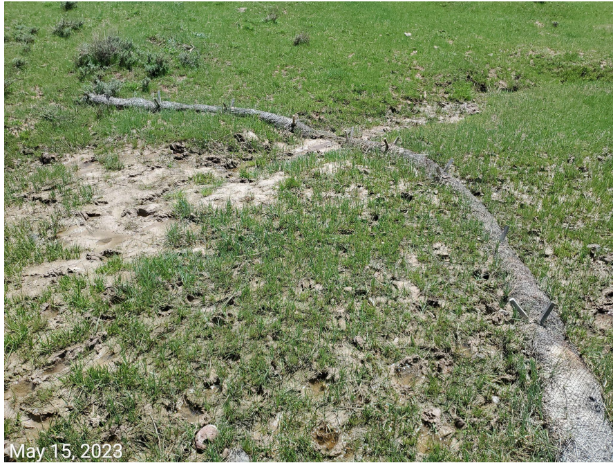
Photo 7: Sediment discharge and deposition from the access road.
