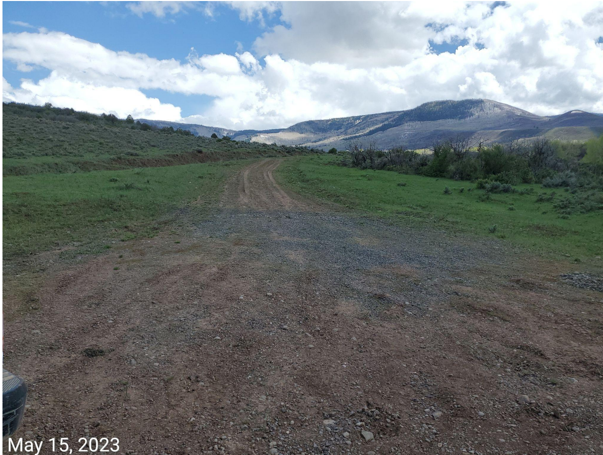
Photo 10: Photo showing the access road has not been reclaimed in accordance with 1004 requirements.
