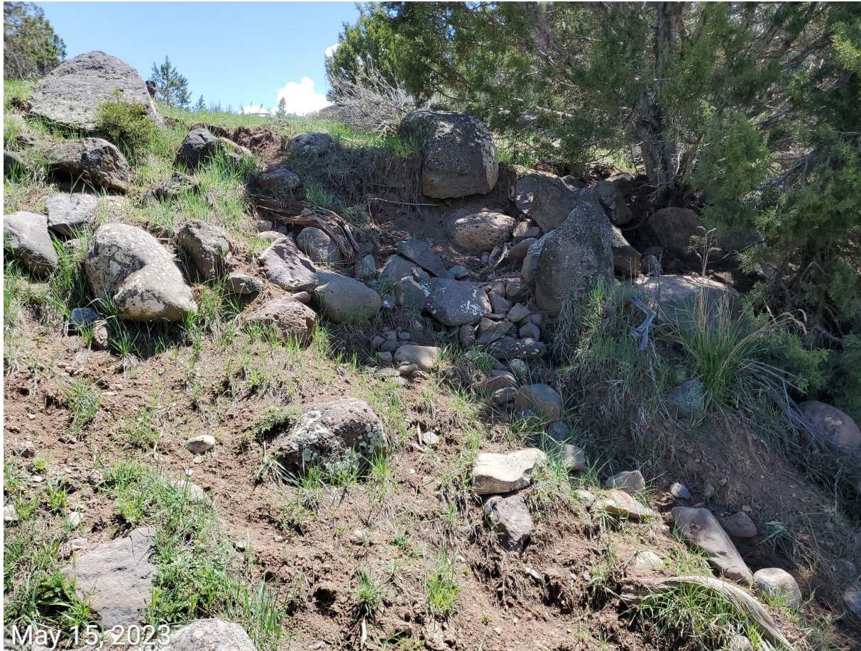
Photo 6: Photo taken from the cut slopes on the northeast end of the Location. Cut slopes lack stabilization; erosion degradation and sediment transport observed.
