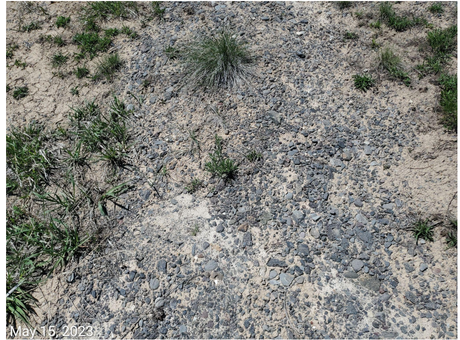
Photo 3: Gravel/Road base material observed remaining on Location.
