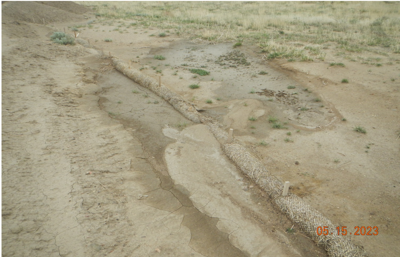
Photo 6. View of wattle which sediment has filled in and overtopped the wattles moving sediment offsite.
