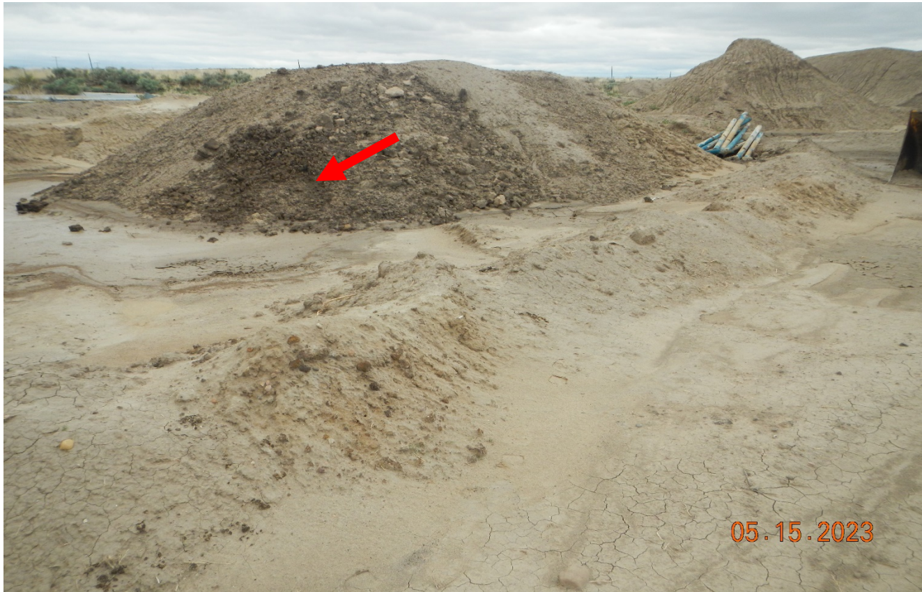
Photo 4. There is no liner observed under the contaminated soils which are not being properly stored. The berms around the material are not compacted or adequately constructed. Contaminated soils need to be removed and properly disposed. Red arrow points to black hydrocarbon soils.
