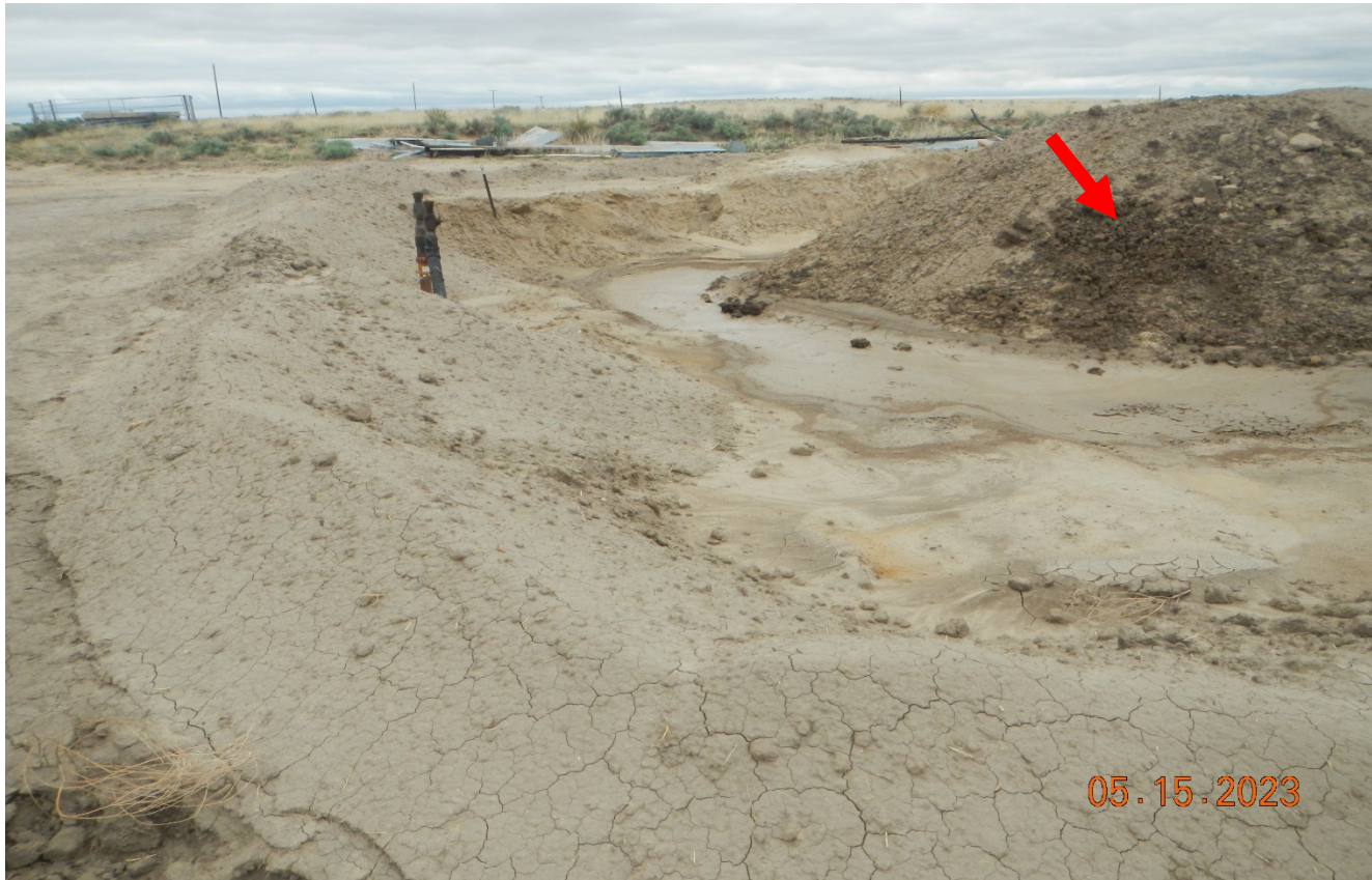
Photo 3. Facing southeast toward the tank battery facility. The tank was removed and soils were excavated in this area. It appears soils have been backfilled into the excavated area where tanks were located. There is still a pile of contaminated material improperly stored at the location. Red arrow points to black hydrocarbon soils.
