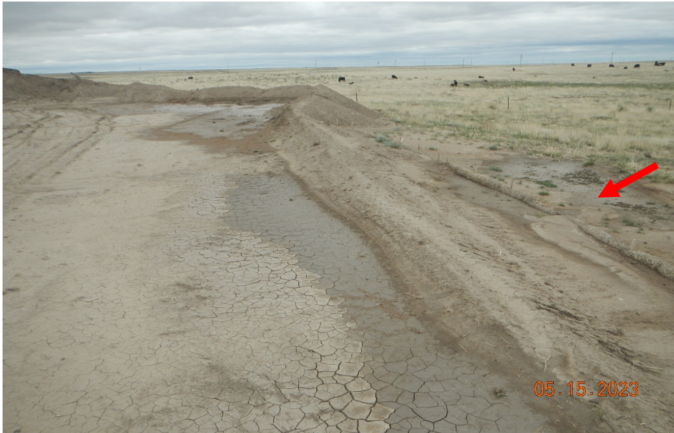
Photo 5. Facing south at the tank battery facility. There is insufficient stormwater controls in this area and the wattles at red arrow has filled in has overtopped the wattles moving sediment offsite.
