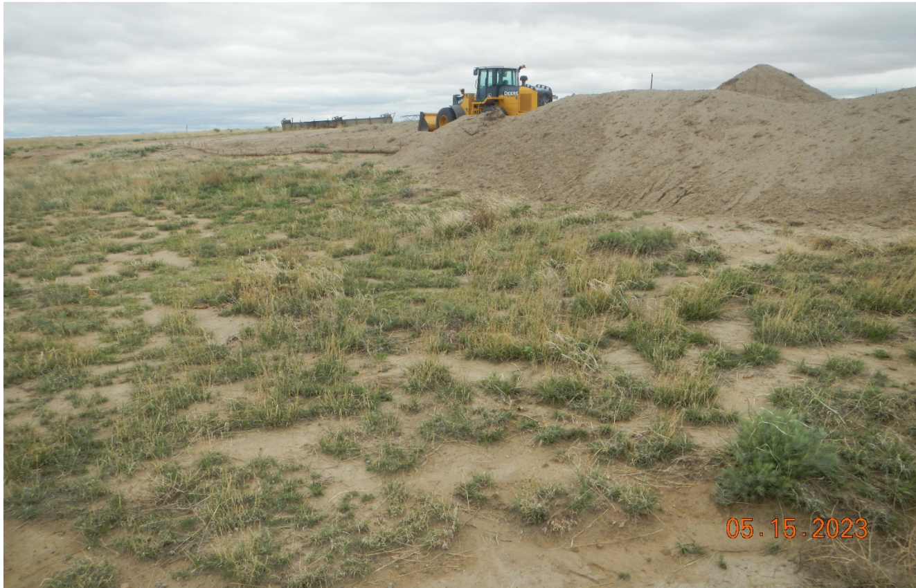
Photo 7. There have been soils brought in and stockpiled at the south side of the location. There is inadequate stormwater BMP's to prevent erosion of the stock piled soil. Previous corrective action was not completed.
