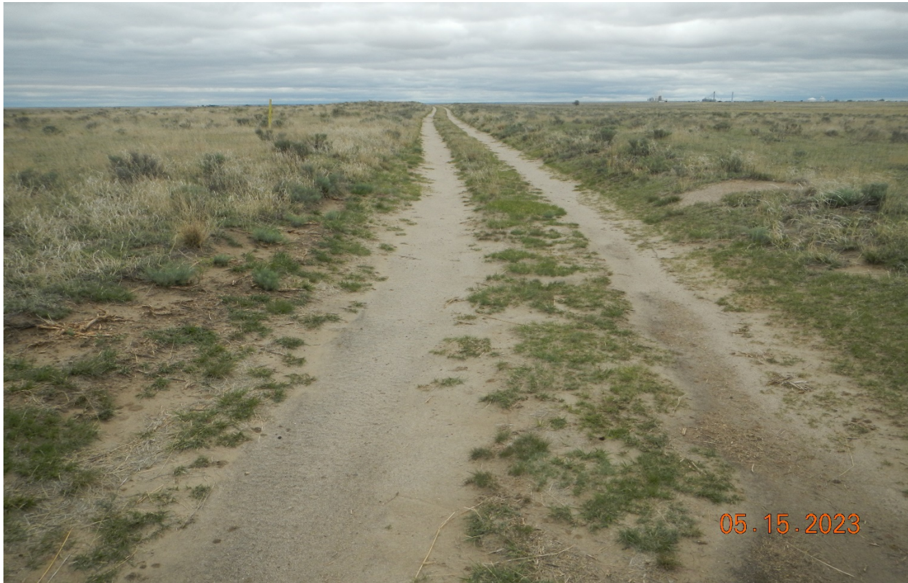
Photo 1. Facing north along the access road. This portion of the road has not been recontoured and reclaimed. Previous corrective action not completed.
