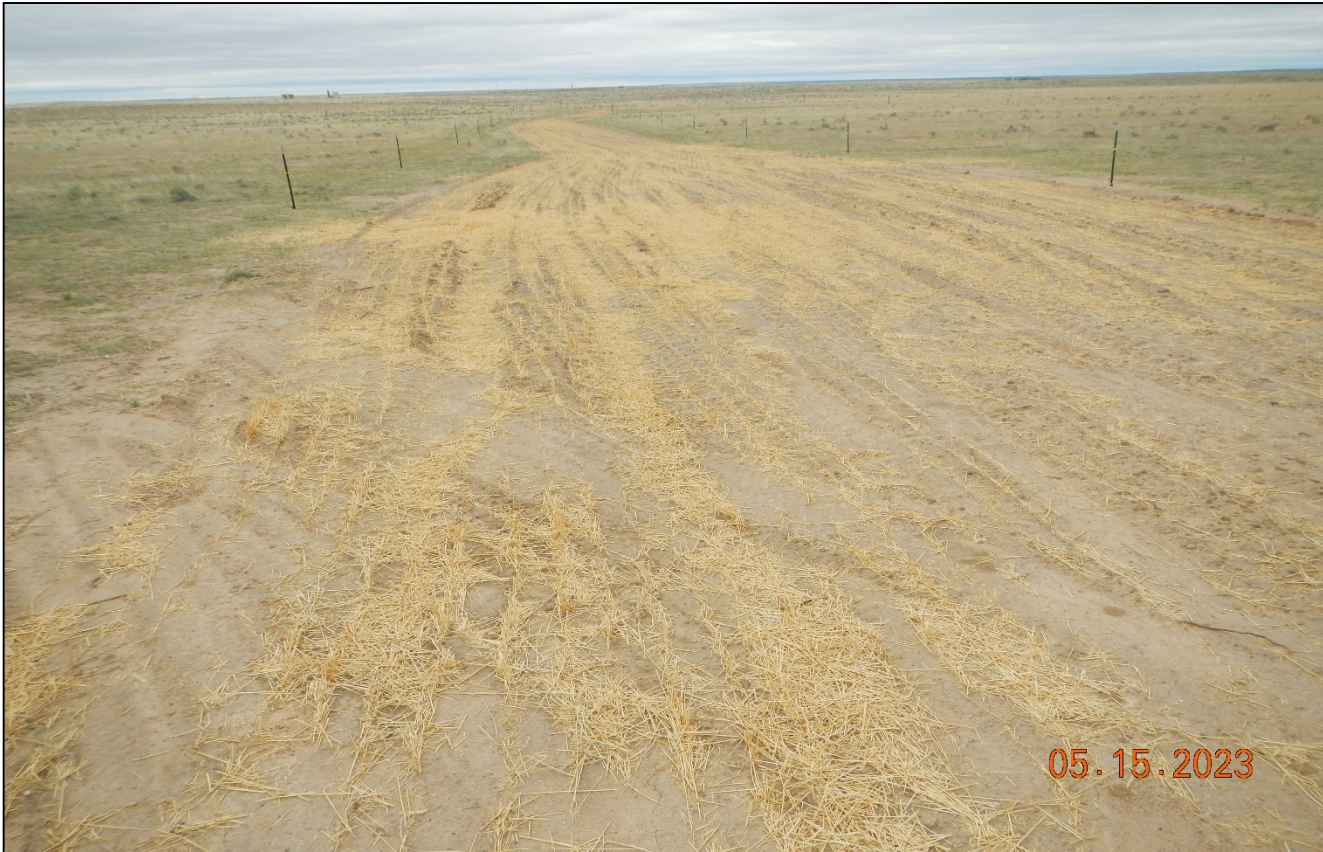
Photo 1. Facing west at the beginning of the access road. The cattleguard has been removed and the road regraded and reclaimed.
