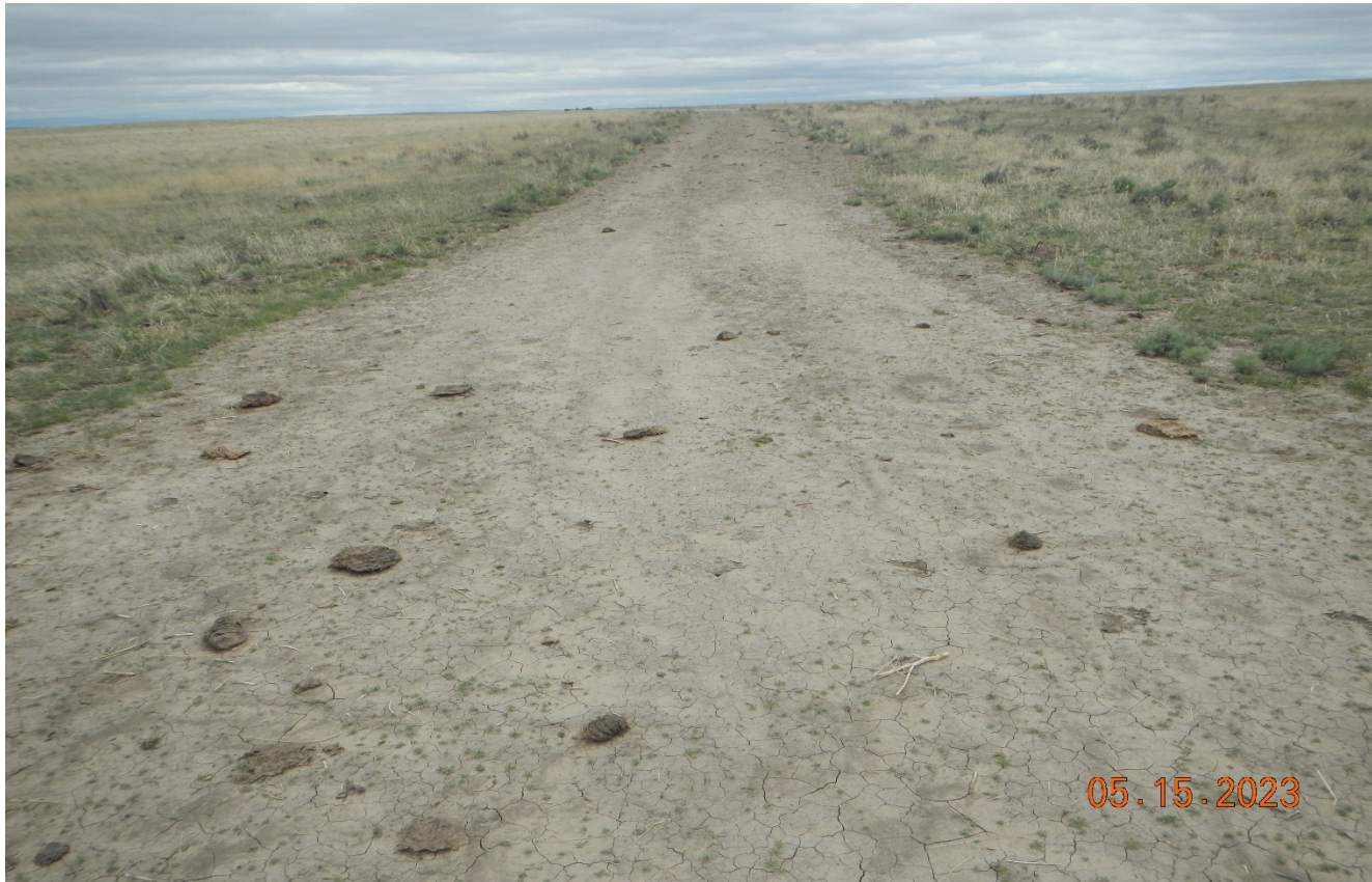
Photo 1. Facing north toward the access road. It appears soil has been hauled in and decompacted but it does not appear that seeding has been completed.
