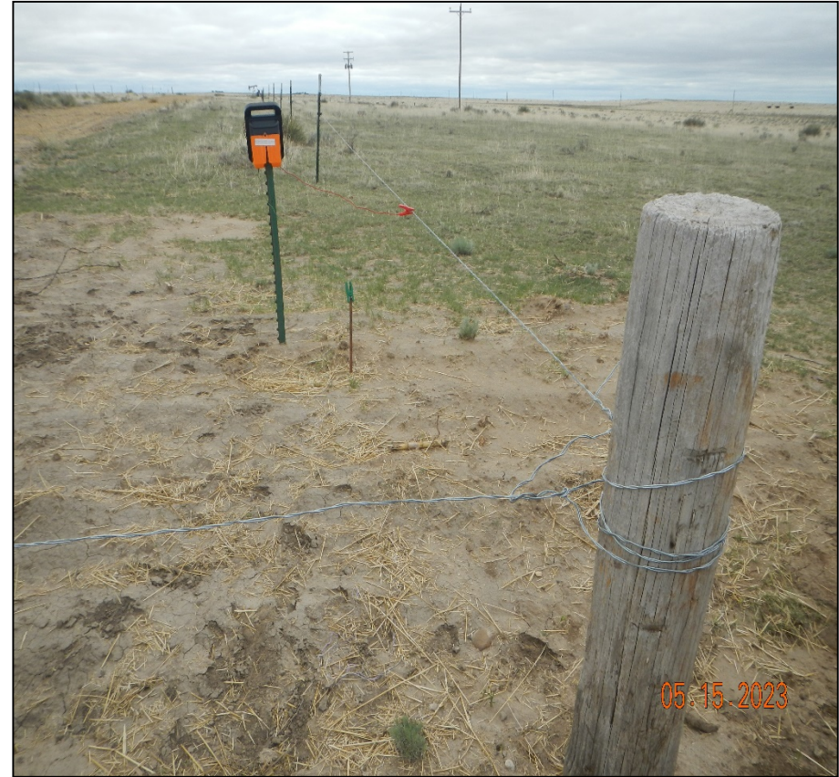
Photo 7. The electric wire does not have any current flow down the line. No insulators were used on the wood posts. Another solar charger should be used for this long stretch of wire.
