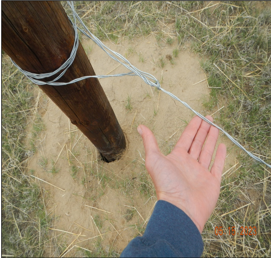
Photo 6. The electric wire does not have any current flow down the line. No insulators were used on the wood posts.
