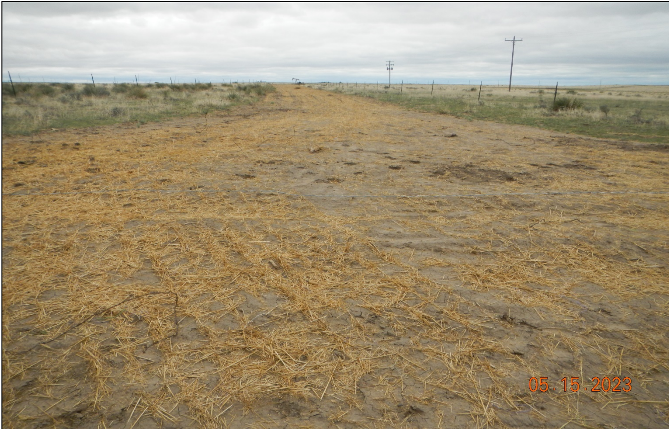
Photo 1. Facing south toward the access road. There has been soil hauled into bring the road back to contour. Soils have been seeded and straw mulched.
