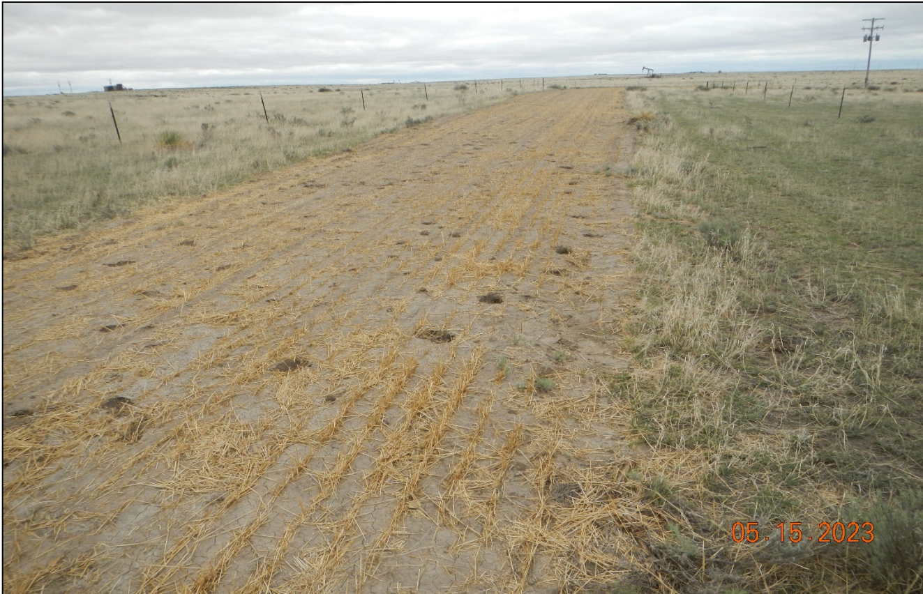
Photo 2. There has been soil hauled into bring the road back to contour. Soils have been seeded and straw mulched.
