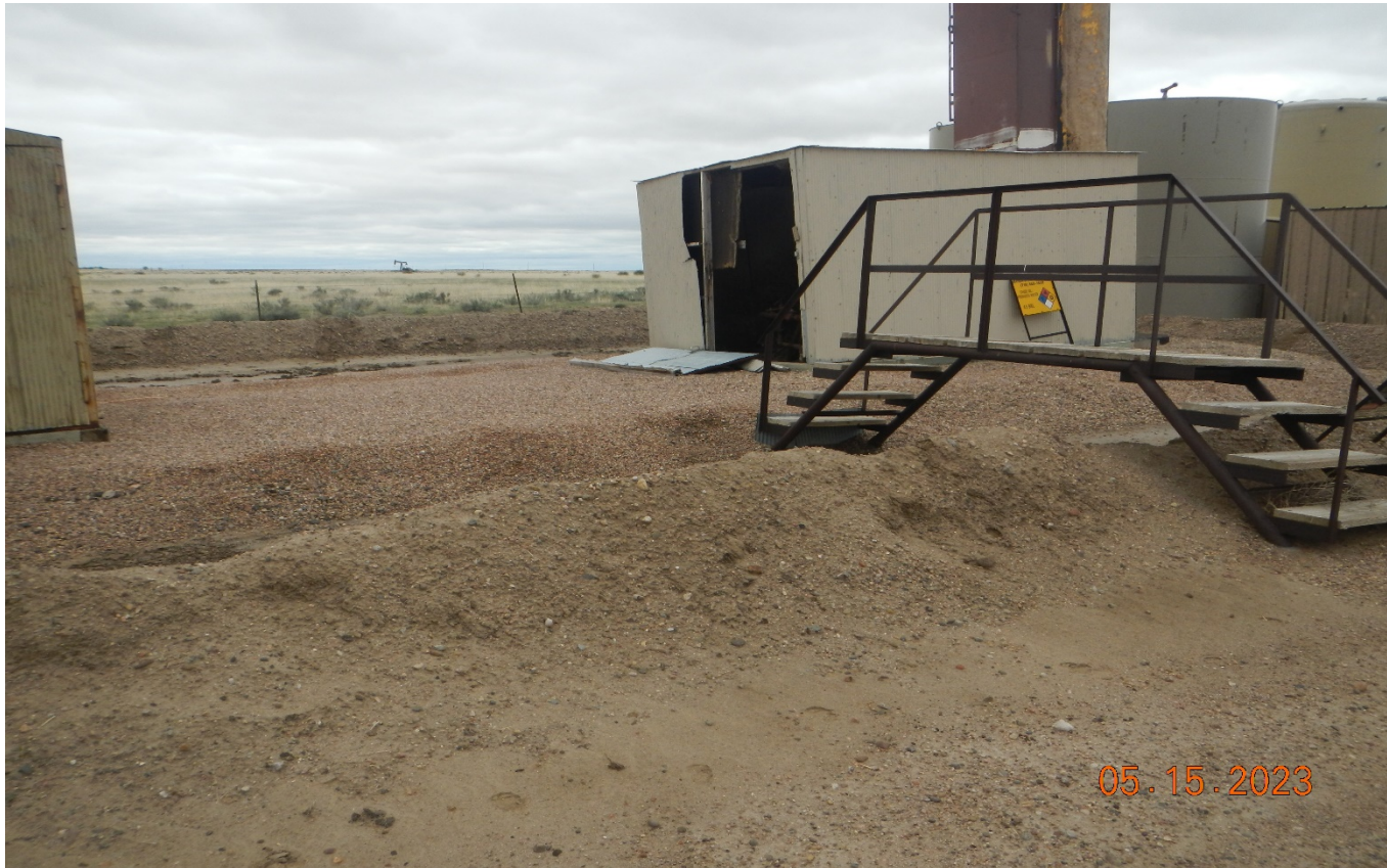
Photo 5. The shed inside the containment battery is not maintained with metal siding laying on the ground.
