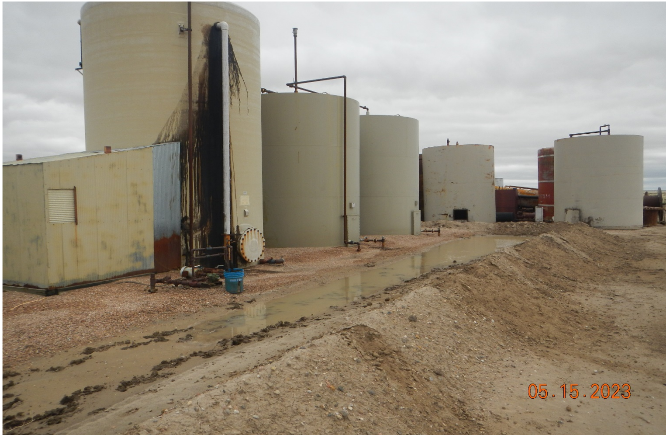
Photo 7. Facing at the back side of the tank battery. There was a spill from the tank which needs to be cleaned up. The blue bucket needs to be emptied and disposed of any oil.
