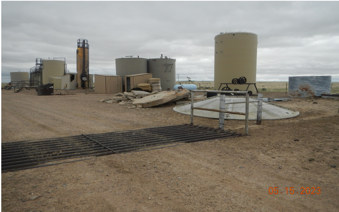
Photo 9. Facing southeast toward the PYLES offsite tank battery and storage yard. There is concrete debris and a broken bottom of a tank among other debris and equipment that must be removed per Rule 606 & 1003.a.
