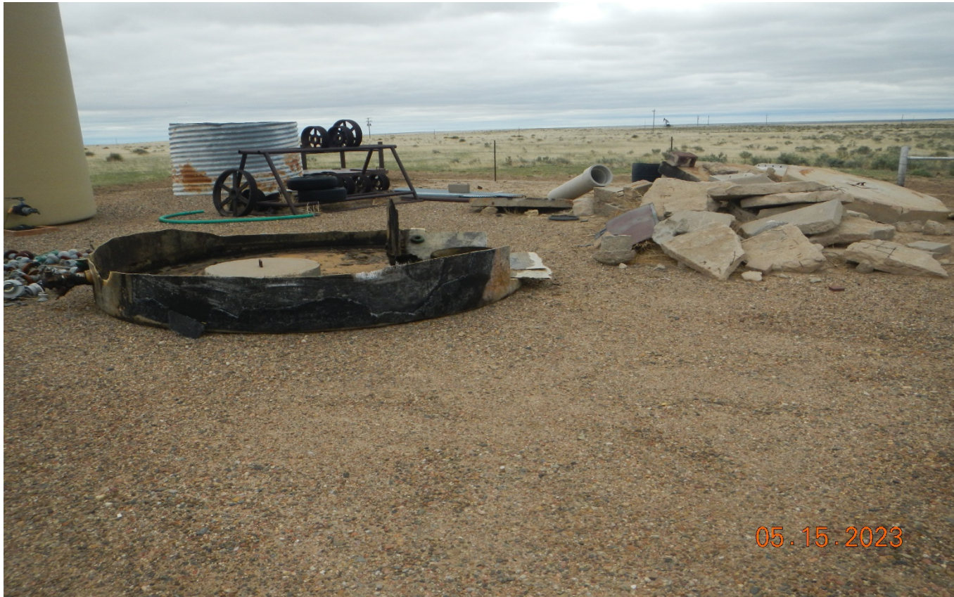
Photo 8. Facing toward the southwest side of the location. There is concrete debris and a broken bottom of a tank among other debris and equipment that must be removed per Rule 606 & 1003.a.
