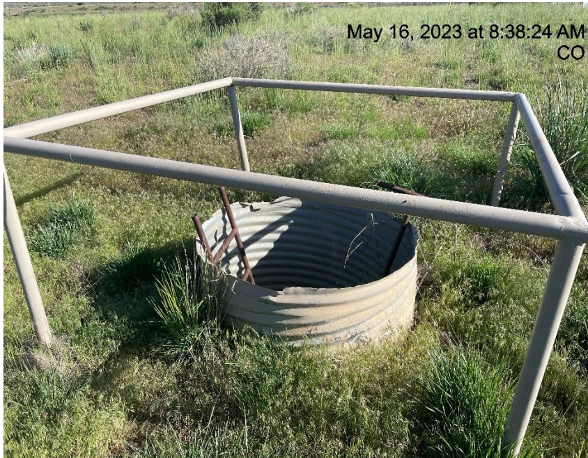
Photo # 7867 Open cellar/wildlife hazard (Cellar is off the north side of lease road approximately 1/10 of a mile from location)
