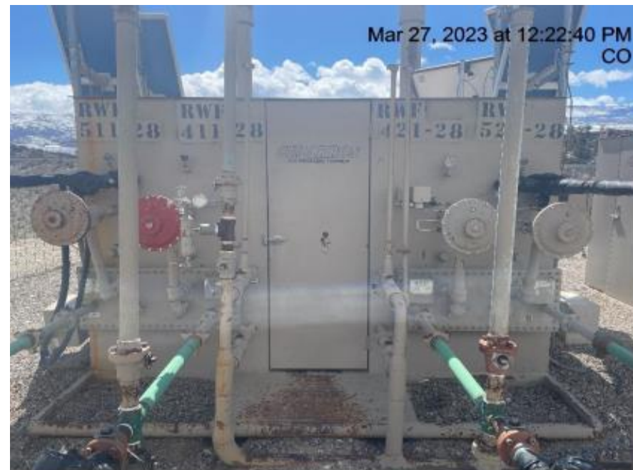
Photo # 3407 From inspection 708900173 conducted on 03/27/2023 Meter calibration info not conspicuously posted
