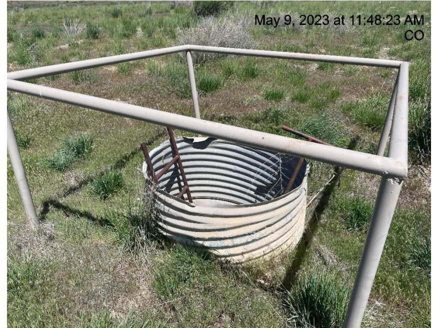
Photo # 7360 From inspection 708900441 conducted on 05/09/2023 Open cellar/wildlife hazard (Cellar is off the north side of lease road approximately 1/10 of a mile from location)
