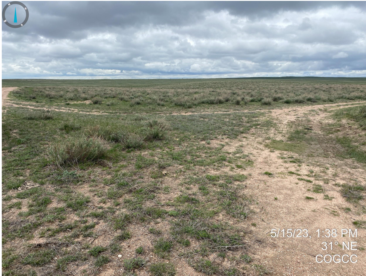
Photo 1. It does not appear the access road has been reclaimed with the presence of road base material and evidence that the road has not been contoured/graded to reflect adjacent areas (e.g. cut slopes pictured in next photos).
