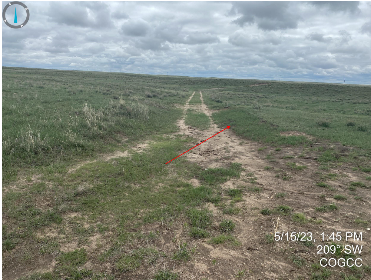
Photo 8. Access road will need to be reclaimed, including but not limited to, removing road base, decompacting, and contouring/grading to reflect adjacent topography/areas.
