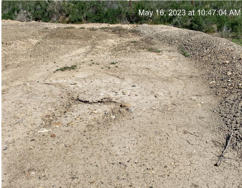
Berm erosion and sediment migration
