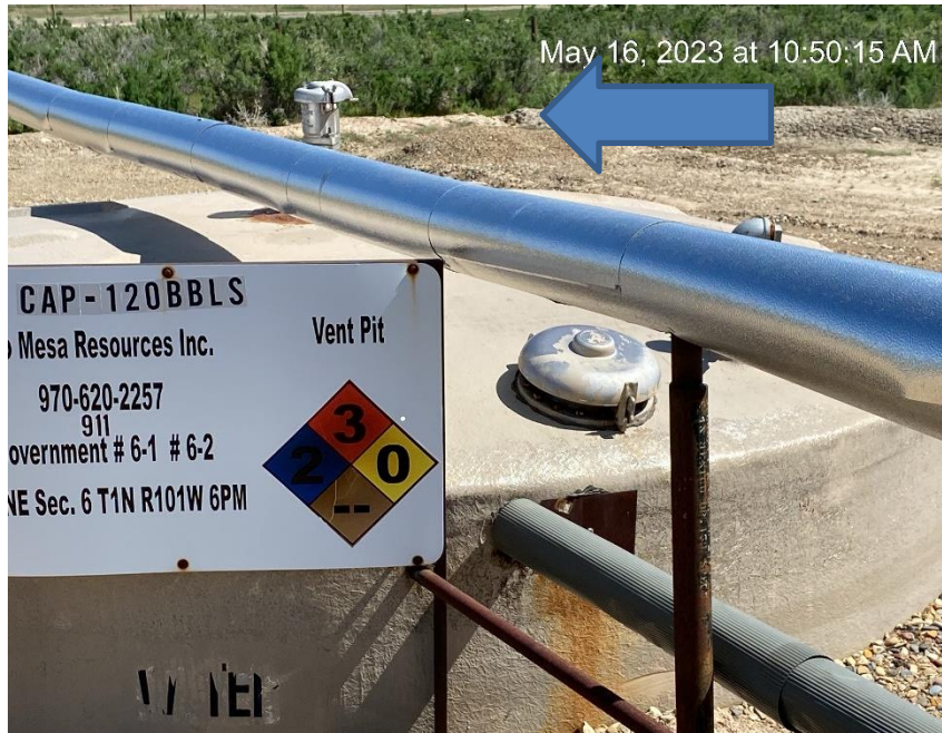
Buried vent tank without sufficient berm
