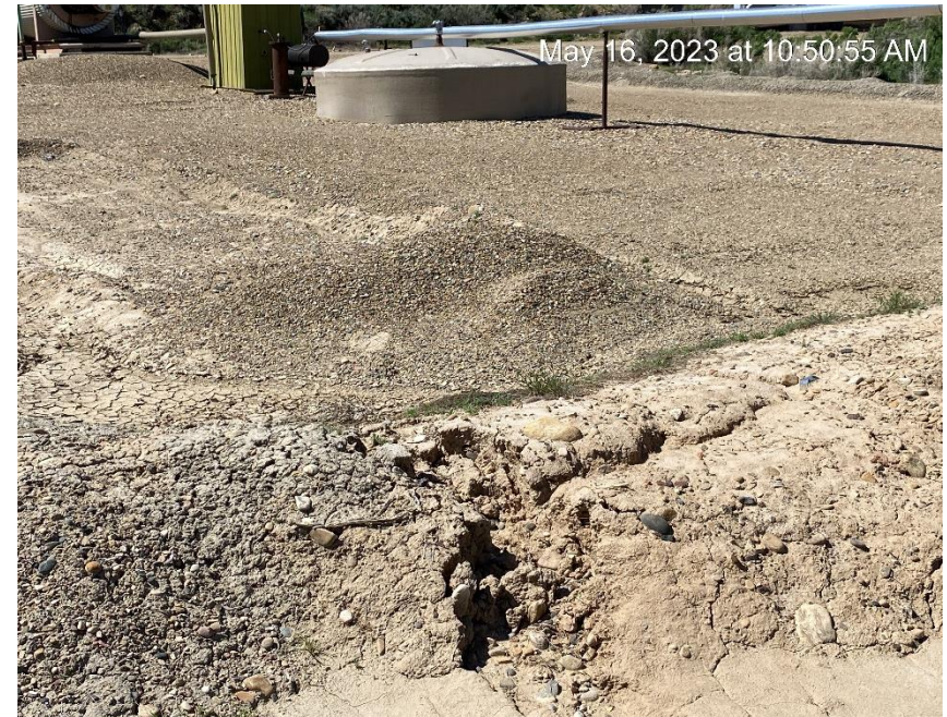
Downhill berm insufficient. No containment.
