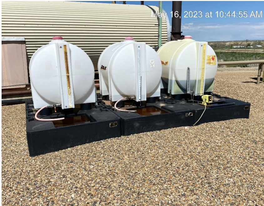
Left and middle tanks without pumps. Unused equipment. Containments full.
