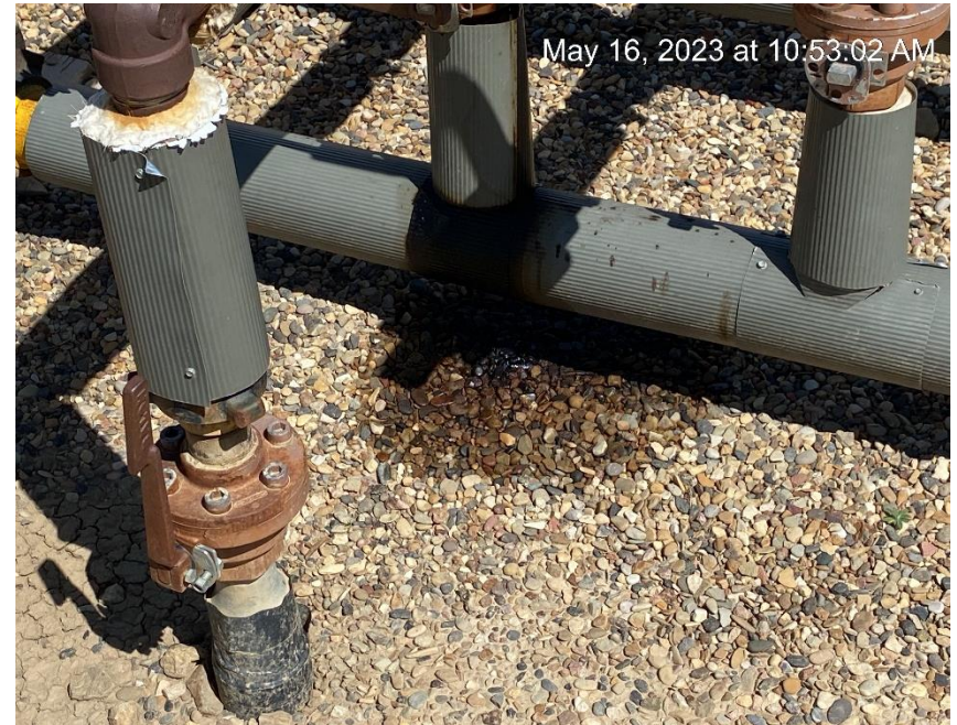
Oil leak and stained soil
