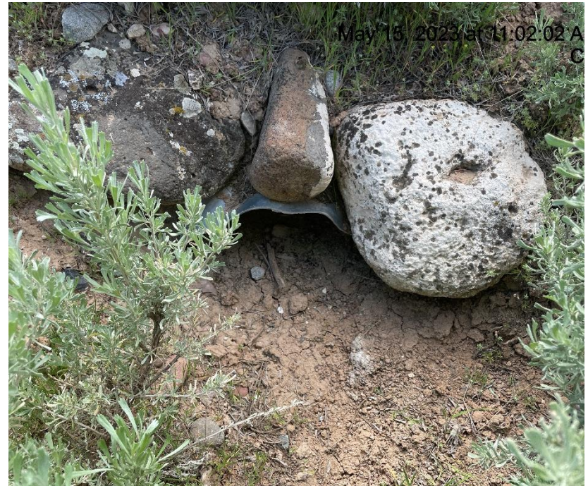
Photo # 7809 Culvert needs maintenance (Culvert is near entrance to location)
