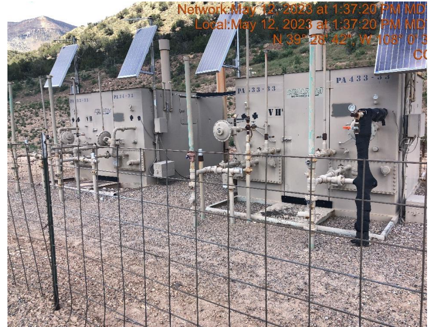
Photo #9975 Calibration cards not conspicuously posted.
