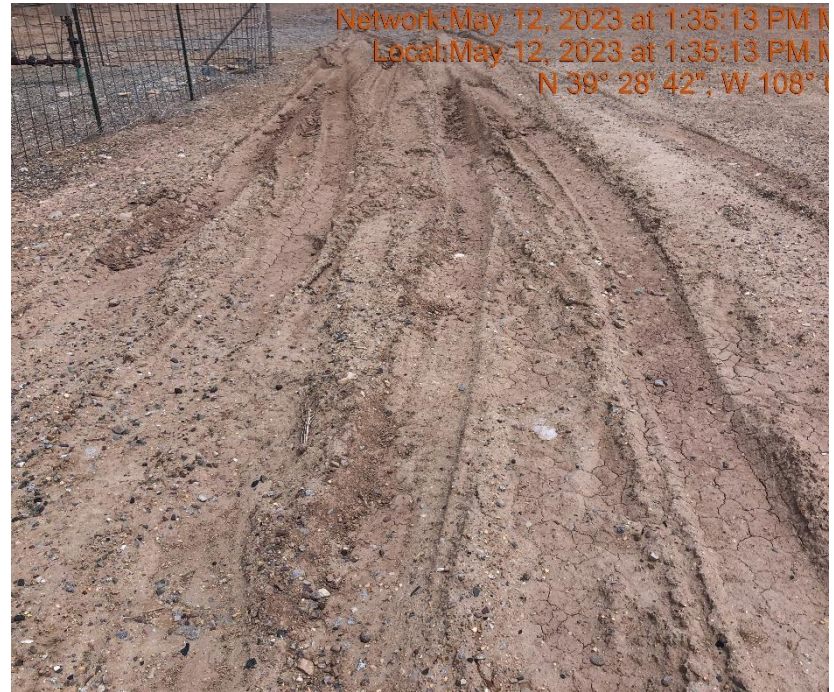
Photo #9967 Location lacks stabilization.
