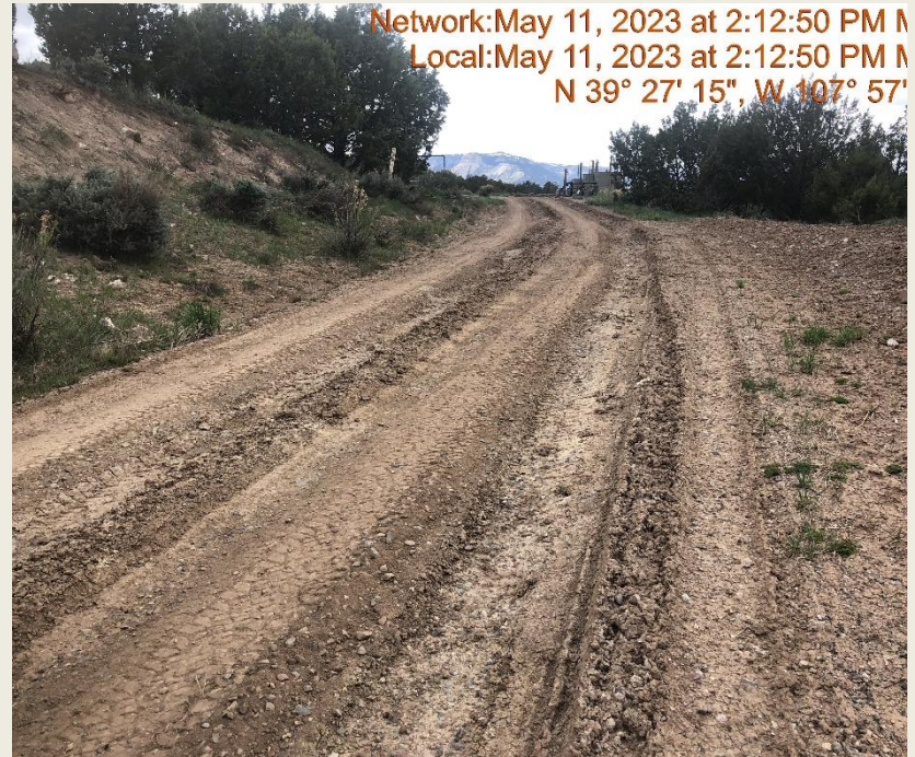
Photo #9955 Access road lacks stabilization.
