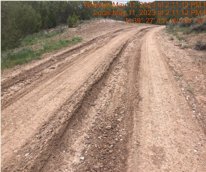
Photo #9952 Access road lacks stabilization.
