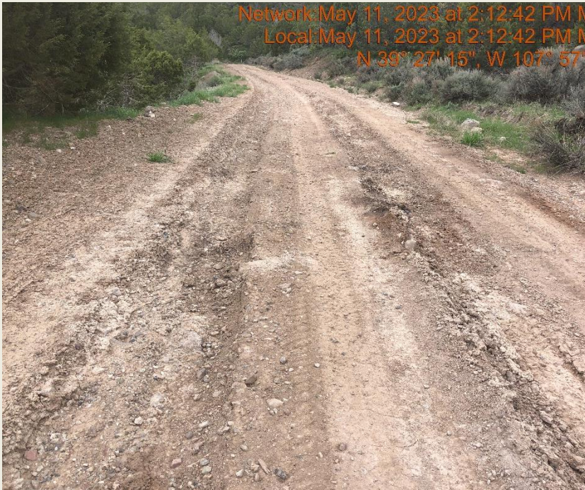
Photo #9954 Access road lacks stabilization.
