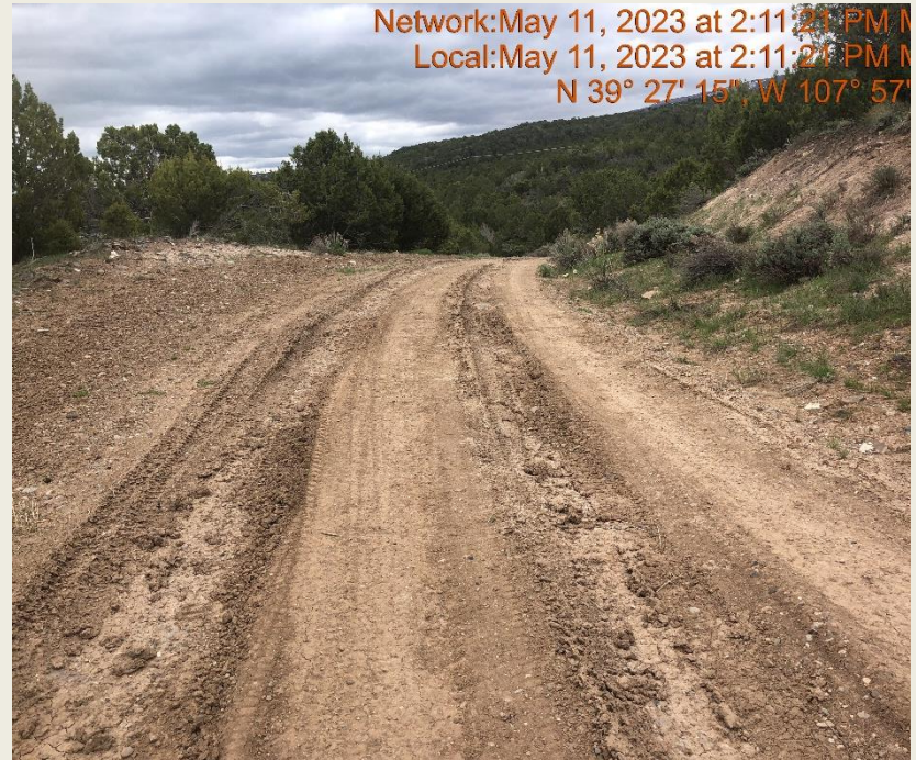
Photo #9953 Access road lacks stabilization.
