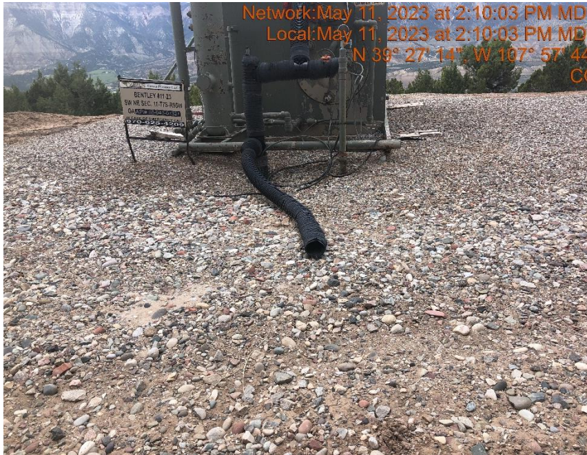
Photo #9946 Flowline heating insulation open ended and not capped.
