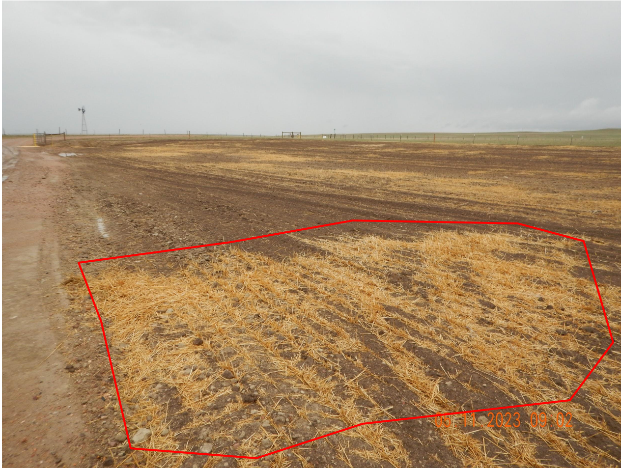
Photo 5. Photo taken from the southern interim reclamation area, facing East. Photo illustrates an area highlighted in red. This area is an example of COGCC's expectation of soil stabilization that shall be reflective throughout the interim reclamation areas, including the topsoil stockpile.
