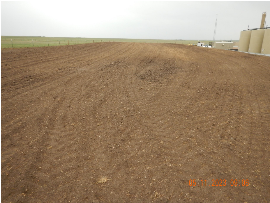
Photo 6. Photo taken from the topsoil stockpile, facing East. Photo illustrates the topsoil stockpile which has been seeded; however, the topsoil stockpile lacks soil stabilization.
