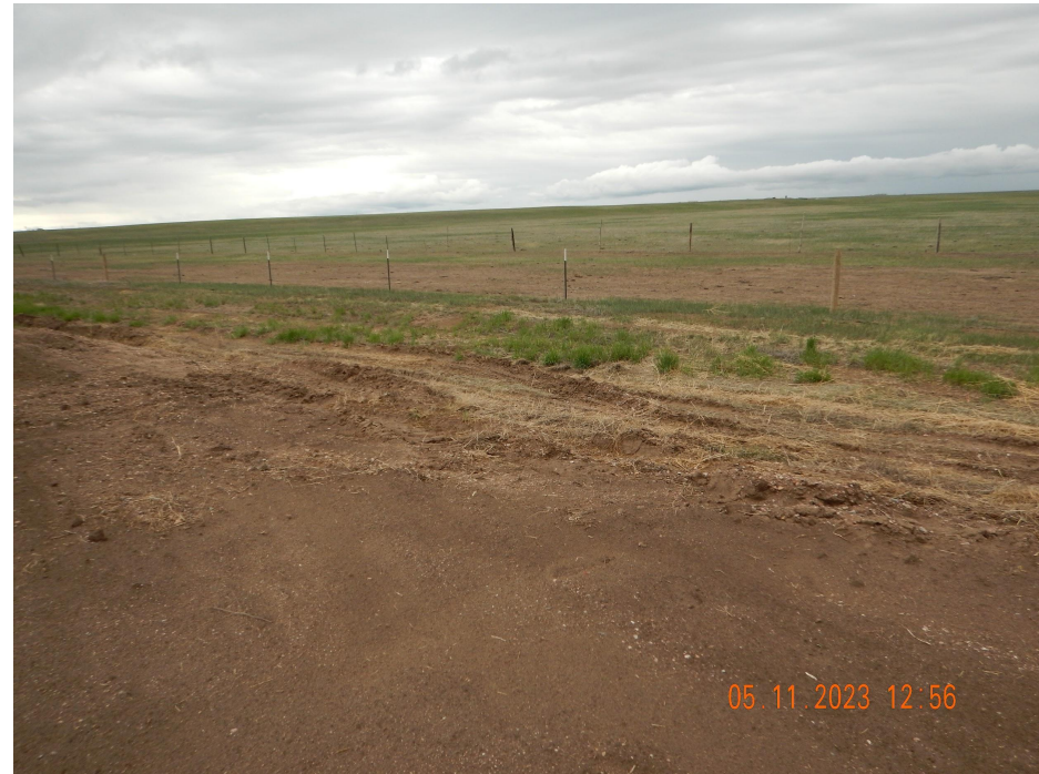
Photo 2. Photo taken from the southeastern location, facing Northeast. Photo illustrates the what appears to be the straw mulch that blew away in a dust storm.
