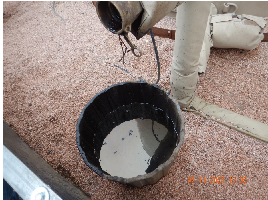
Photo 8. Photo taken from the facility location. Photo illustrates an open bucket with oil that is missing wildlife protection devices.
