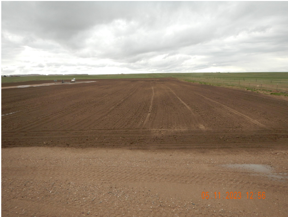
Photo 1. Photo taken from the southeastern location, facing North. Photo illustrates interim reclamation has been performed; however, interim reclamation is not complete due to the lack of soil stabilization. It appears that straw mulch was crimped but blew away in a dust storm.
