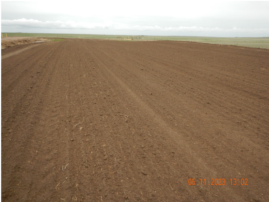
Photo 7. Photo taken from the topsoil stockpile, facing East. Photo illustrates the topsoil stockpile which has been seeded; however, the topsoil stockpile lacks soil stabilization.
