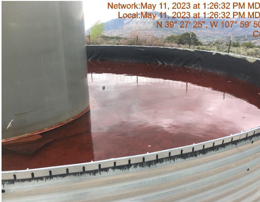
Photo #9941 Secondary containment capacity reduced.
