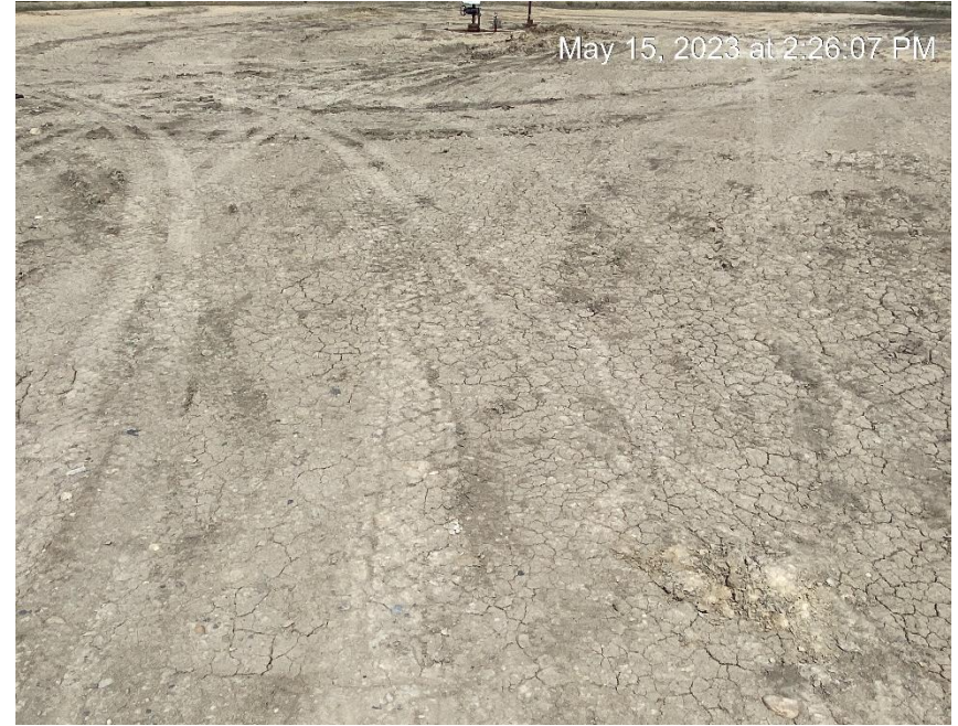
Entrance to location
