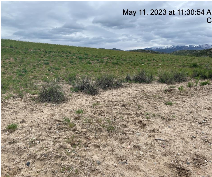
Photo # 7565 Berm & ditch need maintenance
