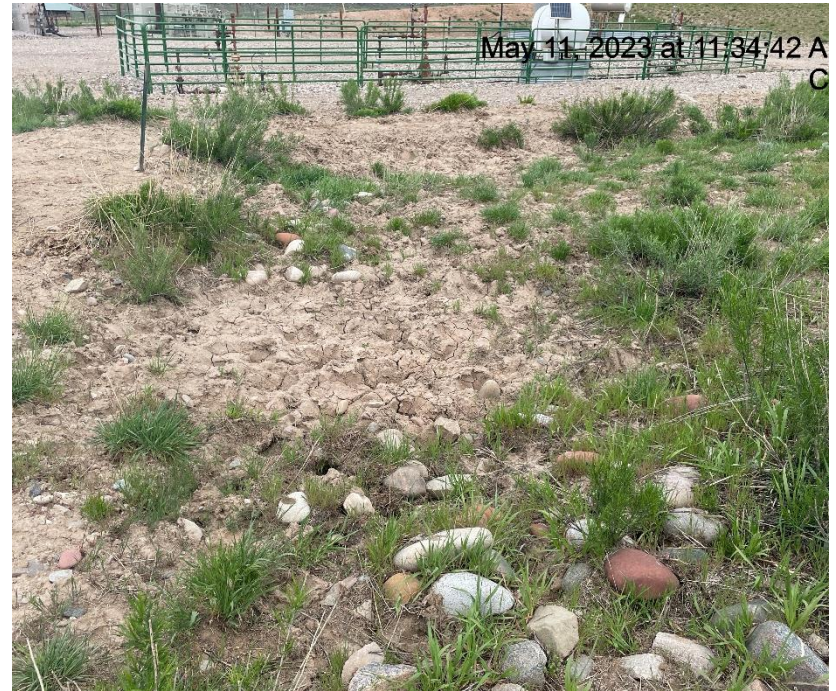
Photo # 7570 Sediment trap needs maintenance
