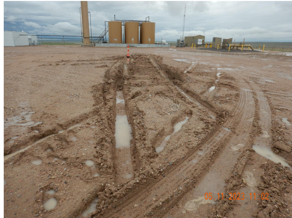
Photo 11. Photo taken from western well location, facing South. Photo illustrates vehicle rutting in need of repair.
