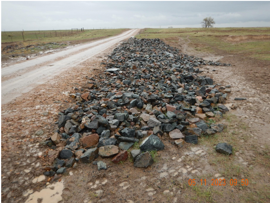
Photo 1. Photo taken from Geary Creek, facing East. Photo illustrates riprap has been imported to stabilize the fill slope into Geary Creek and control stormwater runoff into Geary Creek.
