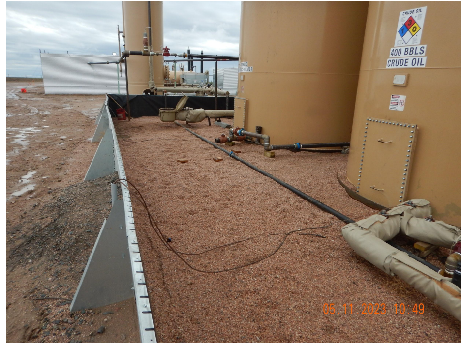
Photo 9. Photo taken from the production area, facing South. Photo illustrates it appears oily waste underneath the load out has been cleaned up.
