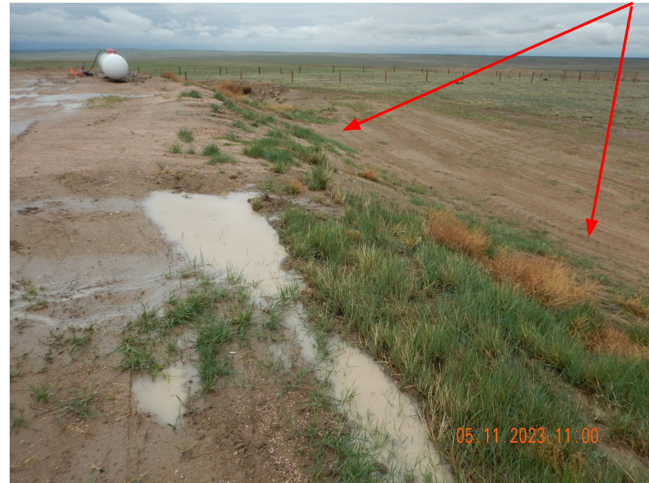
Photo 7. Photo taken from western fill slope, facing South. Photo illustrates the point of sediment laden stormwater discharging off location without a perimeter BMP (red arrows indicating no perimeter BMP).
