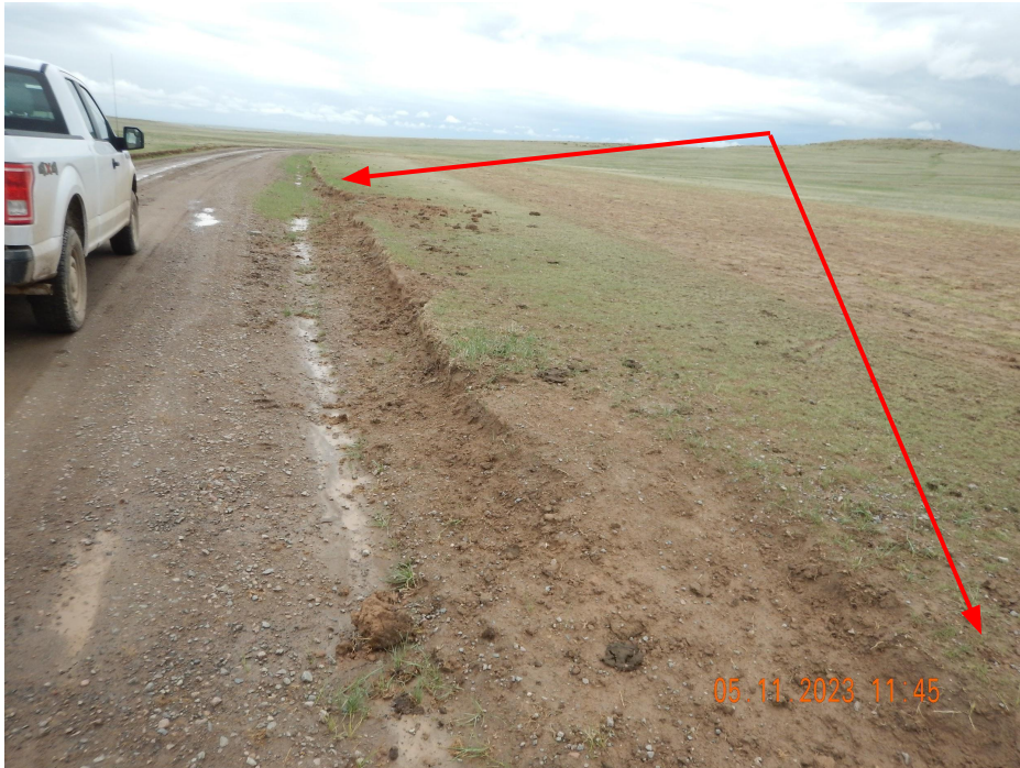
Photo 17. Photo taken from a portion of the access road approximately at the 3.7 mile marker, facing East. Photo illustrates the reclamation of access road repairs have not been completed. Photo illustrates the roadside area has been disturbed during snow removal by Upland.
