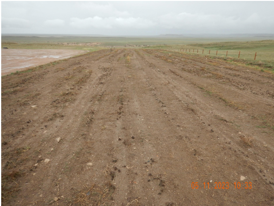
Photo 4. Photo taken from topsoil stockpile, facing West. Photo illustrates the topsoil stockpile has not been stabilized, which was communicated to the Operator back on April 7th. Operator indicated that the topsoil has been reseeded.
