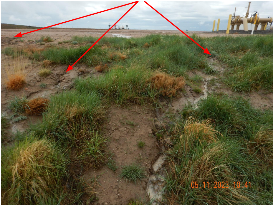
Photo 6. Photo taken from western fill slope, facing East. Photo illustrates sediment laden stormwater discharging off location (red arrows).
