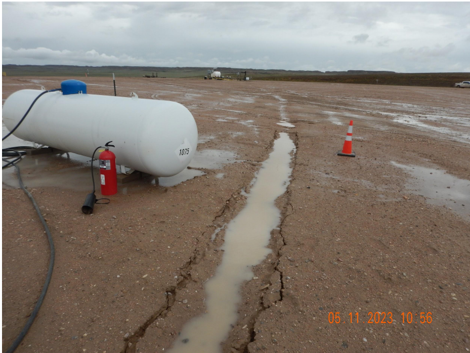
Photo 10. Photo taken from southern well location, facing North. Photo illustrates subsidence along a flowline in need of repair.
