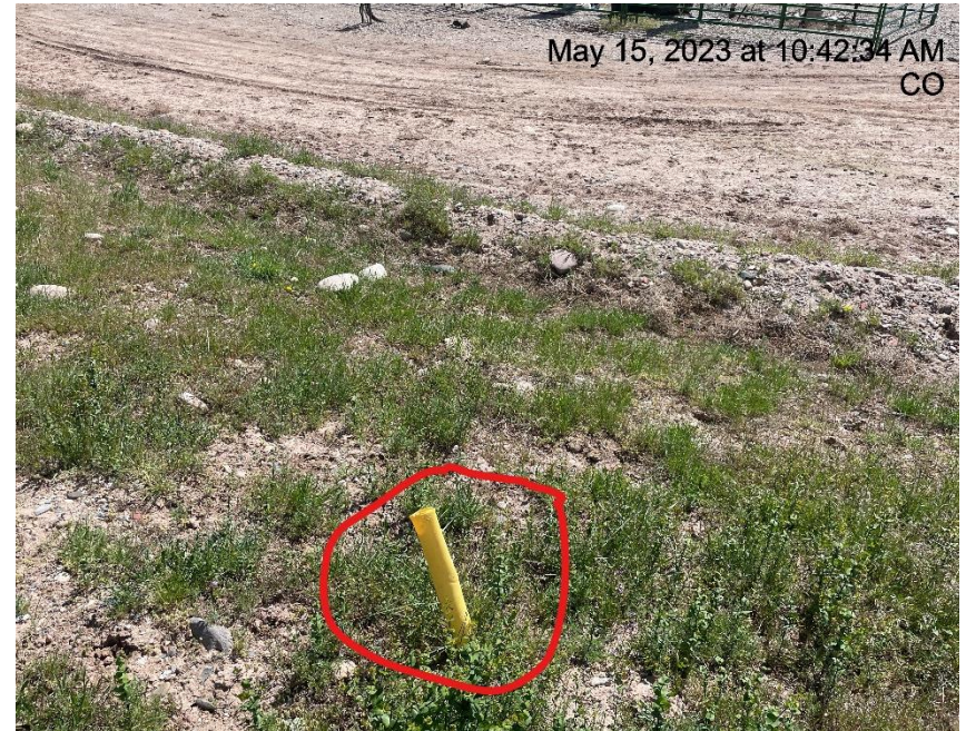
Photo # 7787 Improperly marked deadman
