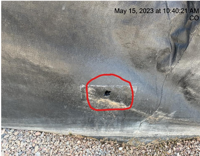
Photo # 7779 Containment liner needs maintenance
