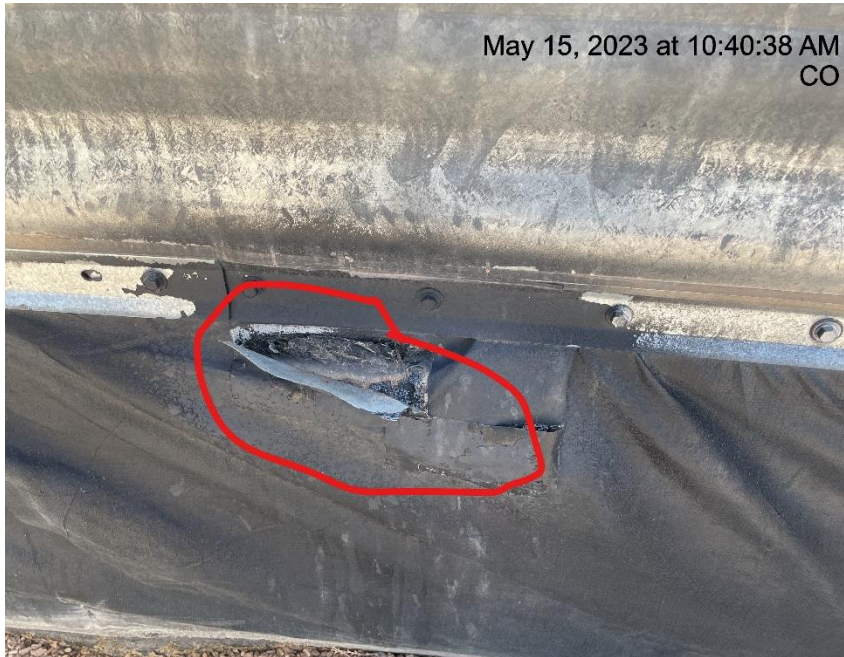
Photo # 7781 Containment liner needs maintenance
