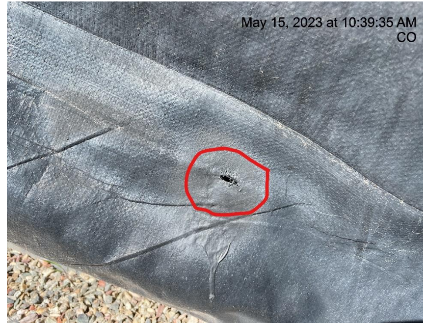
Photo # 7778 Containment liner needs maintenance
