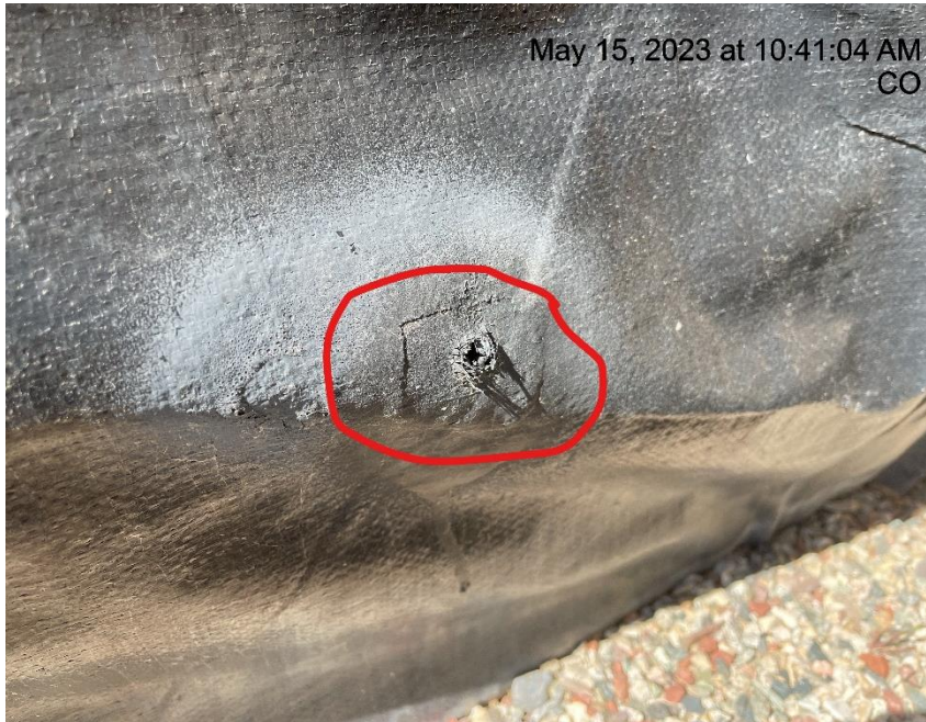
Photo # 7783 Containment liner needs maintenance
